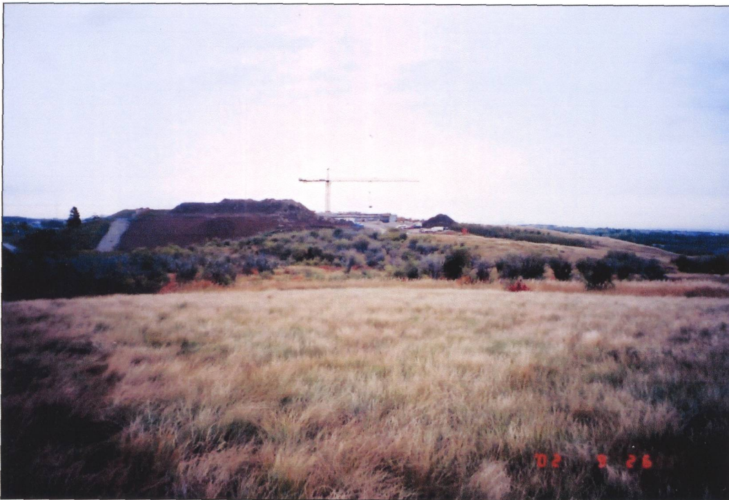
Ungrazed rough fescue grassland (NG) on morainal knoll (foreground) with water reservoir construction (background) – SW quarter of Section 28-25-2w5
