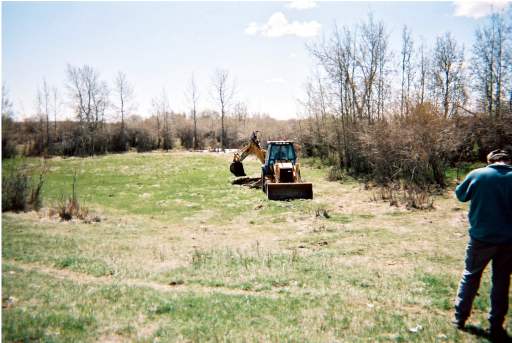
Plate 4. Backhoe Testing Spy Hill Project Area
