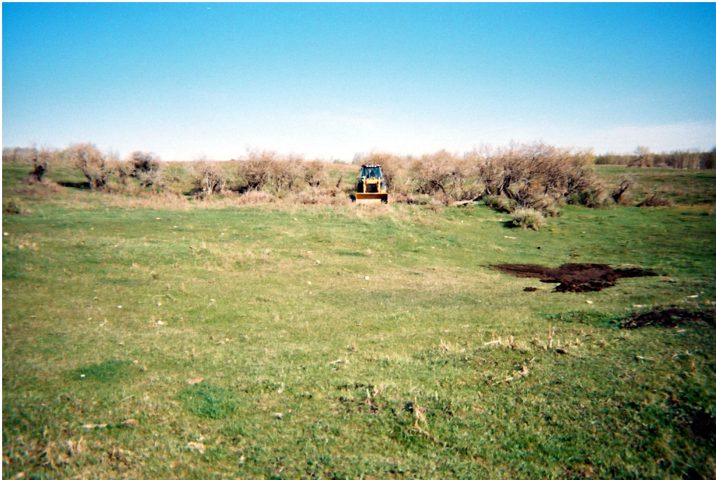
Plate 5. Backhoe Test #2 (View NW)
