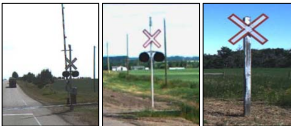
Figure 1- Type 1 (left) and Type 2 (middle) warning systems receive scheduled maintenance while passive warning systems (right) do not.
