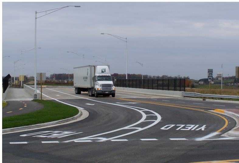
Photo: Ourston Roundabout Engineering
