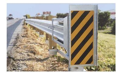
The Extruder Terminal (ET-Plus) is a proprietary, energy-absorbing, gating, tangent end treatment.
