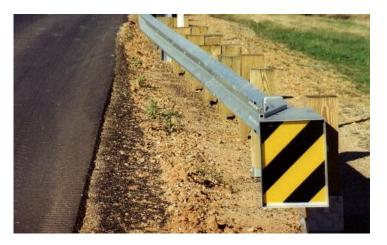
The Flared Energy Absorbing Terminal (FLEAT) is a proprietary, energy-absorbing, gating, flared end treatment.
