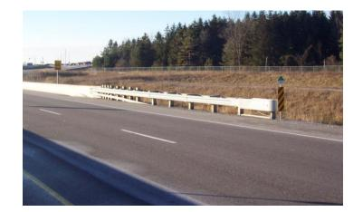
The Crash Cushion Attenuating Terminal (CAT-350) is a proprietary, energy-absorbing, gating, redirective terminal designed to shield narrow hazards.
