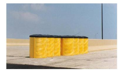
Sand Barrel Systems refer to a family of proprietary, non-redirective, and gating, end treatments.
