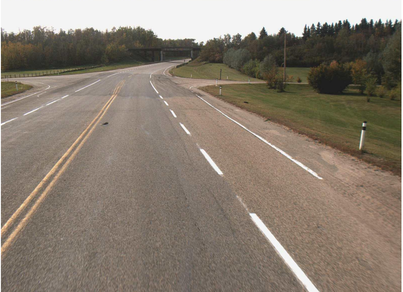
Highway 37:04 – Nelsen Road Intersection, Looking West
