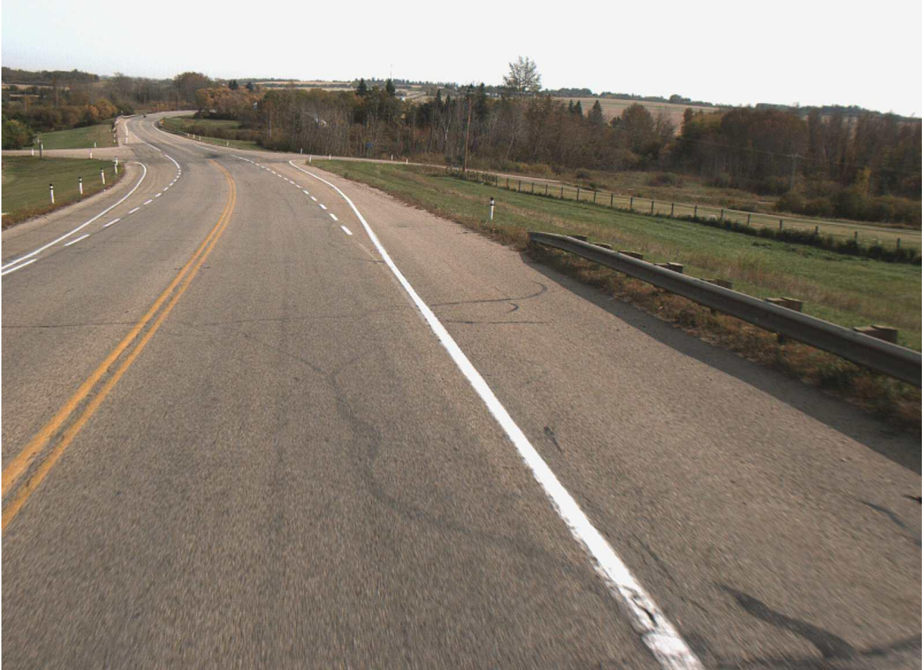
Hwy 37:04 – Nelson Road Intersection, Looking East
