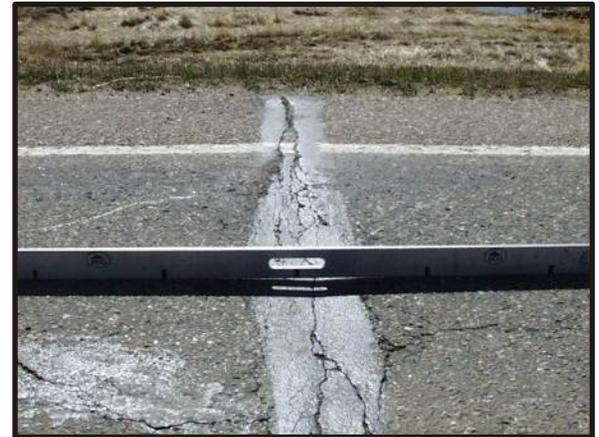
**Extreme Transverse Crack Dipped  $> 6$  mm**
