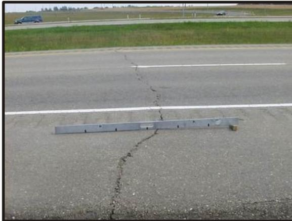
**Moderate to Extreme Transverse Crack Heaved  $> 3$  mm**
