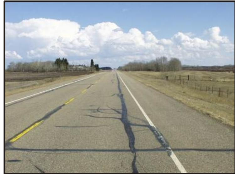
**Centre-of-Paver Crack Located in Outer Wheel path**
