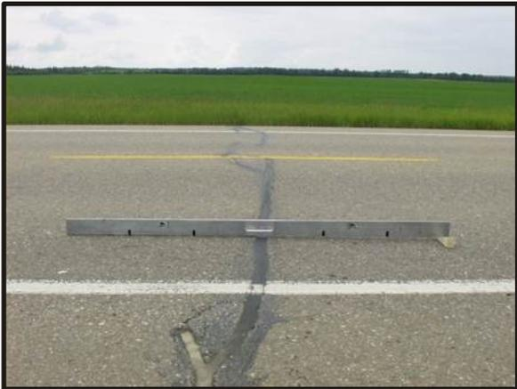
**Repaired Transverse Crack Heaved  $< 3$  mm**
