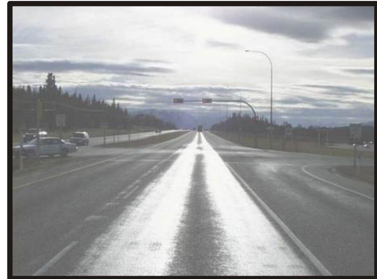
**Extreme Flushing of Seal Coat in wheel paths**
