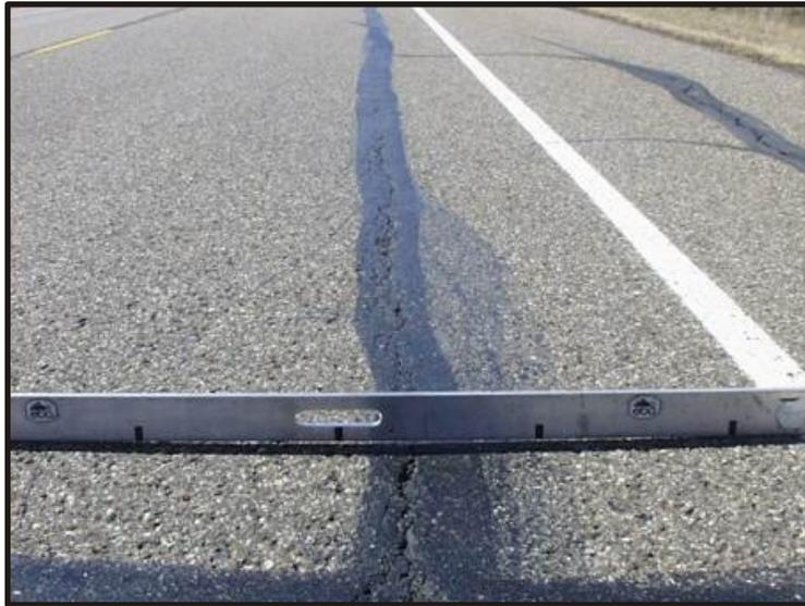
**Moderate Severity Centre-of-Paver Crack**
