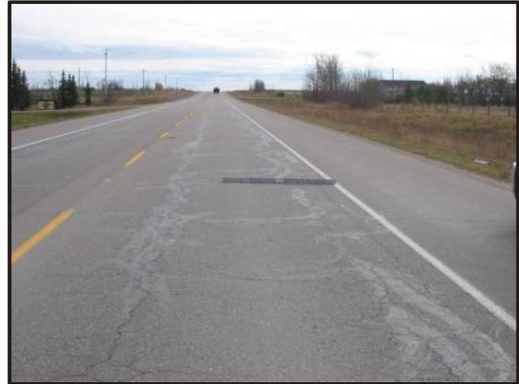
**Extreme Severity Longitudinal Fatigue Cracks**
