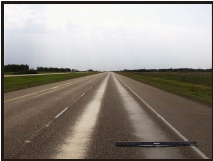
**General Pavement Structure Compaction Rutting**
