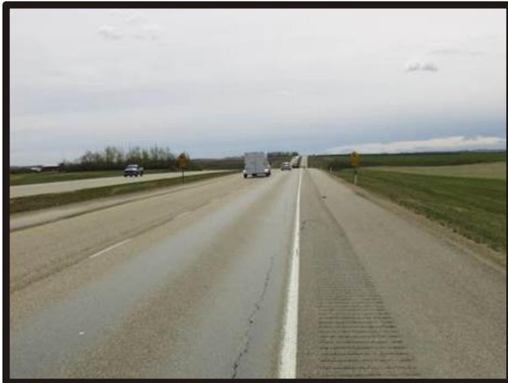
**Slight to Moderate Flushing of Seal Coat in wheel paths**
