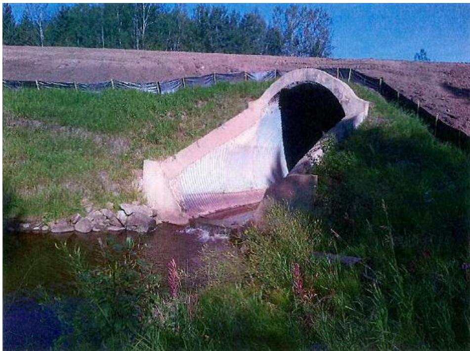
Viewing Culvert Outlet
