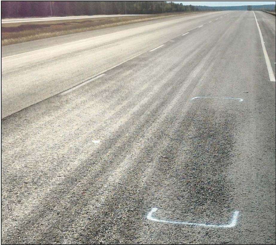
Photograph 8 – Moderate (bordering on Severe) Segregation
