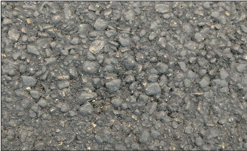
Photograph 9 - Moderate Segregation (bordering on Severe) (Close-Up)
