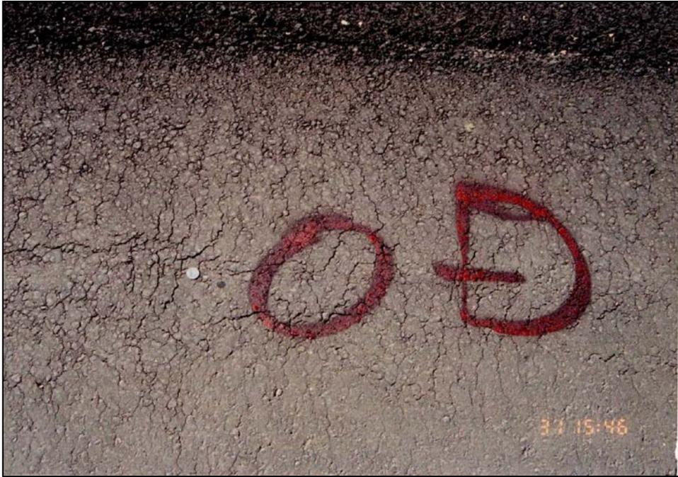
Photograph 17 - Obvious Defect (Hairline Cracking)
