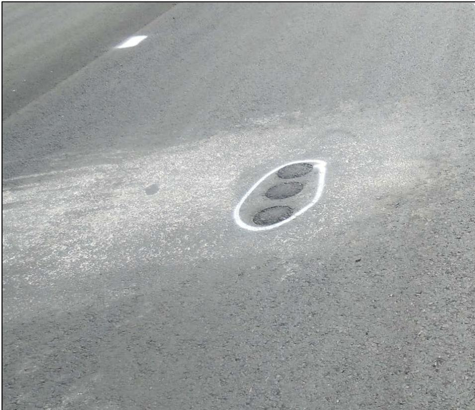
Photograph 16 - Obvious Defect (Improperly Repaired Core Holes)
