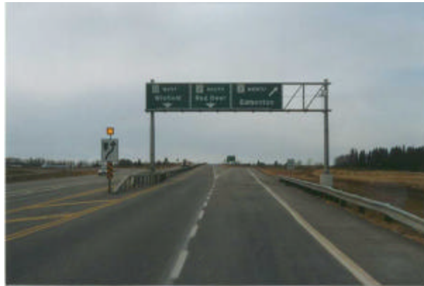
Start of Guardrail Outer Lane
