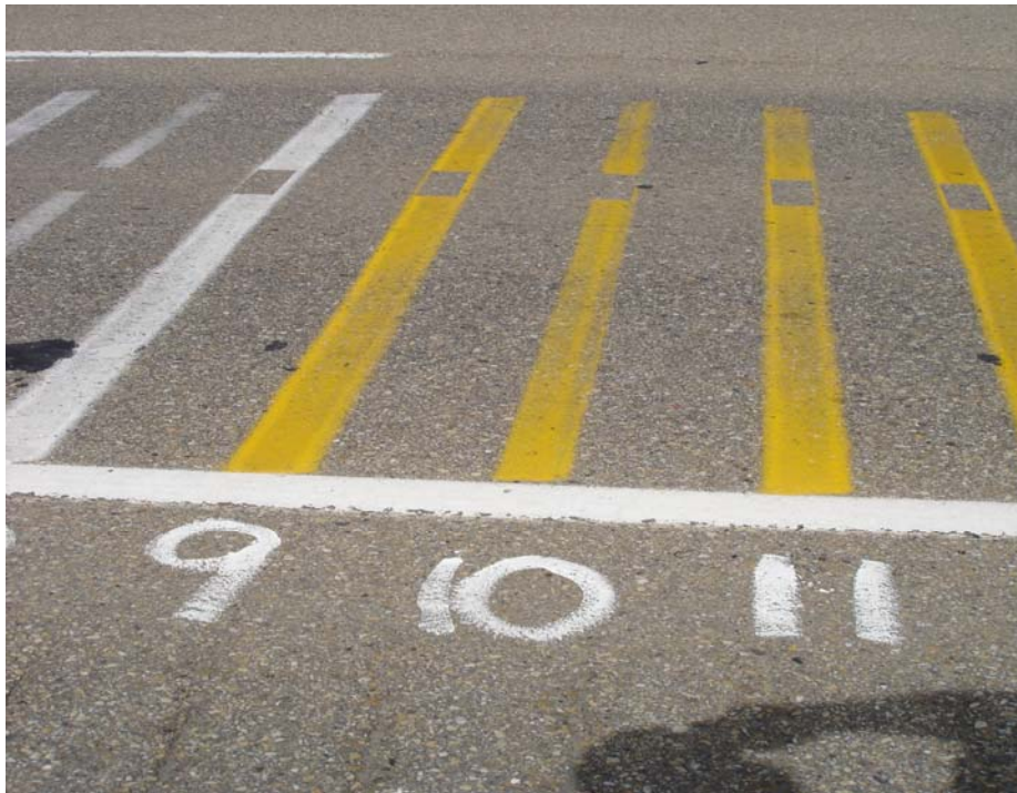
Yellow paint, line #9 – 15mil, line #10 – 12mil and line #11 – 13mil The 12mil line (#10) is almost transparent. The 13mil line (#11) is performing better.
