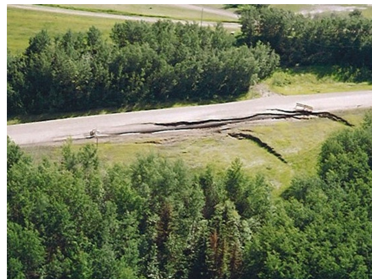
Photo 1. Aerial view of Hines Creek (PH4) Landslide
