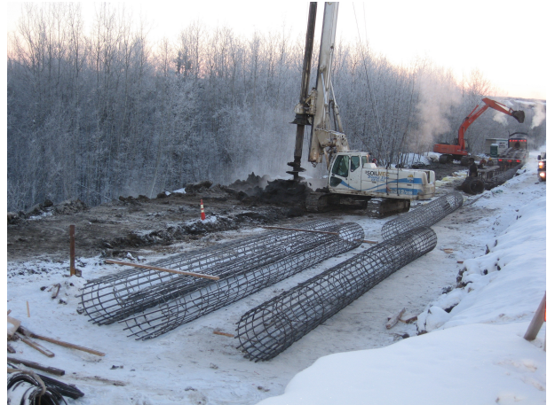
Photo 2. Pile Wall Construction (late January 2008)
