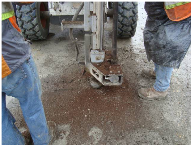
Figure 6. Muskeg blown out of borehole during construction
