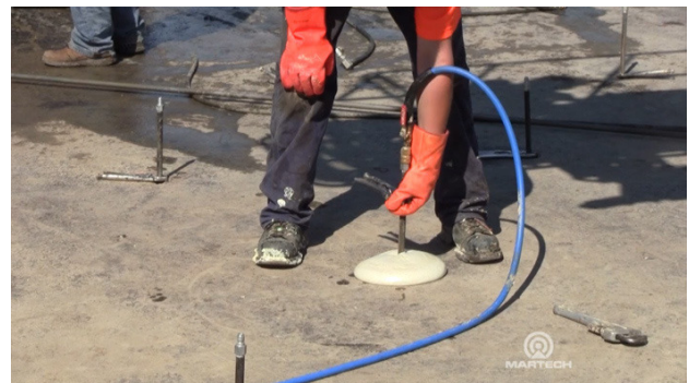
(b) The finish of one foam pile injection
