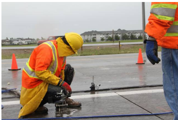
Figure 9 Measuring device to monitor the rise of the concrete panel
