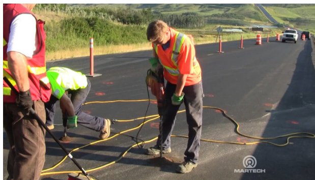
Figure 3. Drill penetrating through 4 feet of pavement structure
