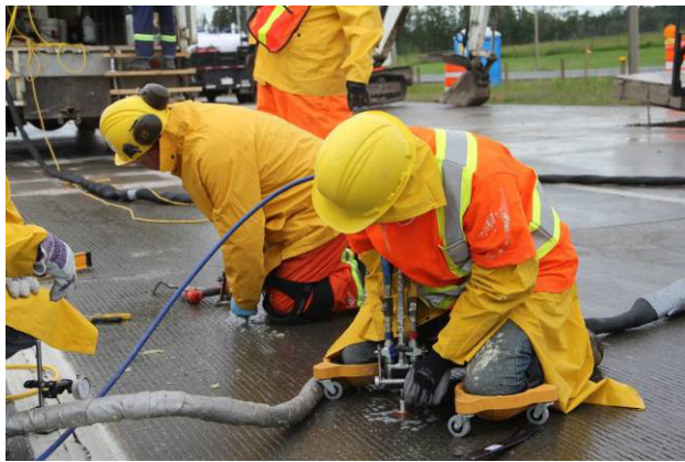
Figure 8 Double injections method to evenly distribute lifting force
