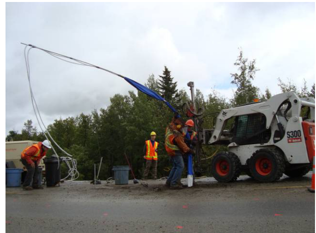
Figure 7. Grouting assembly with tremies, guiding conduit and three-tier sleeve bags
