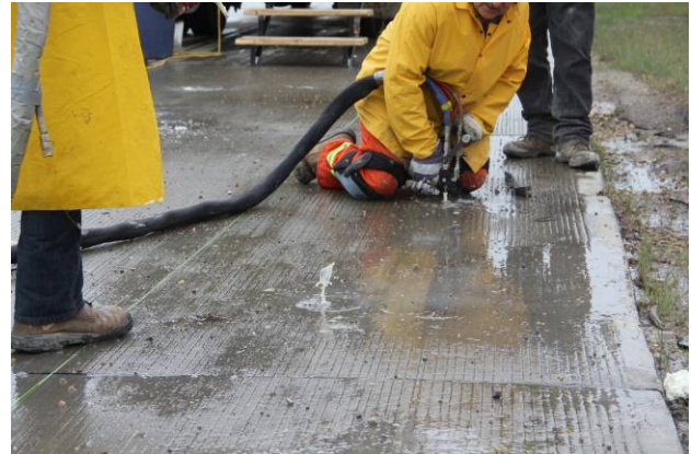
Figure 10 Moisture and water were chased out by expansive polyurethane
