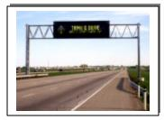
and timely traveller information is provided to the media (e.g. commercial radio). Use of existing dynamic message signs (DMS) in the corridor is also enhanced through the traveller information database and the deployment of additional DMS is recommended in the Red Deer area to improve dissemination of road and weather condition information, particularly in the event of a highway closure.
