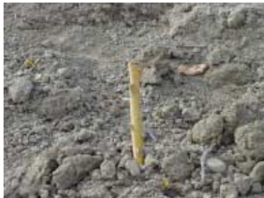
South slope where live stakes and wattles are installed
