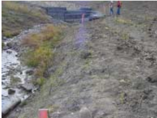
South slope where live stakes and wattles are installed
