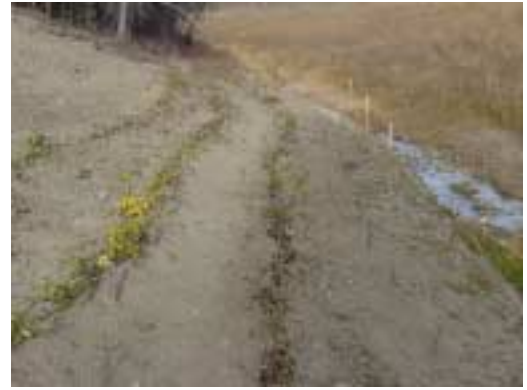
Three rows of willow wattles were installed
