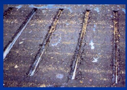
Hairline cracking of pavement at rolled in rumble strips
