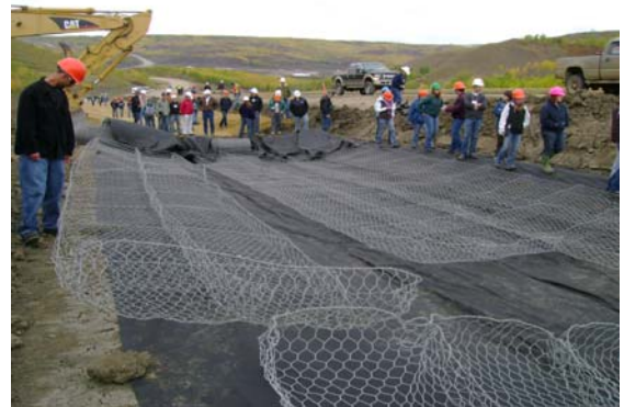
Gabion Mats and Site Tour
