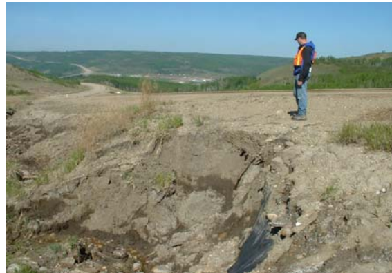
Severely Eroded South Highway Ditch
