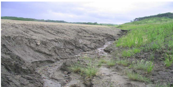
Severely Eroded South Highway Ditch
