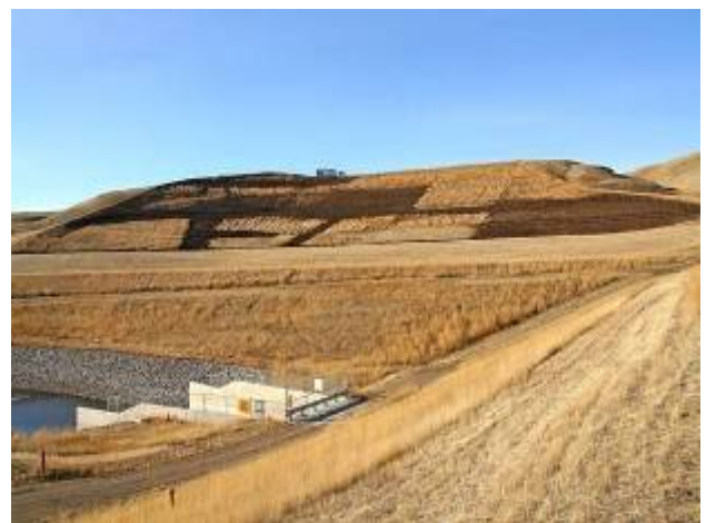
Completed compost berm and blanket (Nov 2008)
