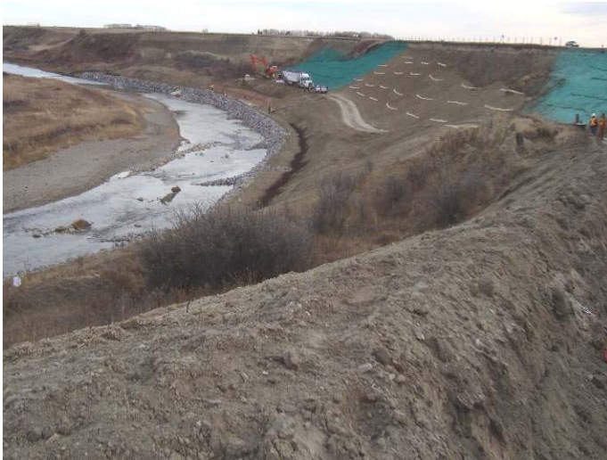
Photo 2: Landslide and river training bioengineering remedial measures implemented at the site, view looking South (November, 2008)
