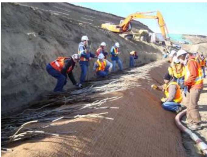
Photo 3: Workshop participants placing willow stakes for brush layering (November, 2008)
