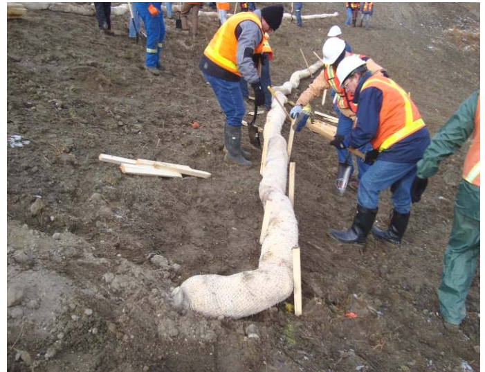
Photo 4: Workshop participants securing coconut fibre rolls on slope (November, 2008)
