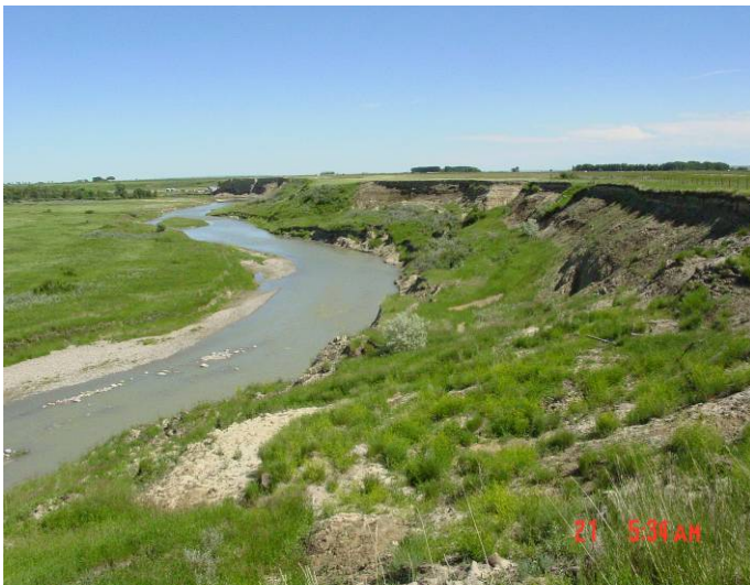
Photo 1: Retrogressive landslides at Willow Creek prior to remedial bioengineering measures, view looking South (June, 2008)
