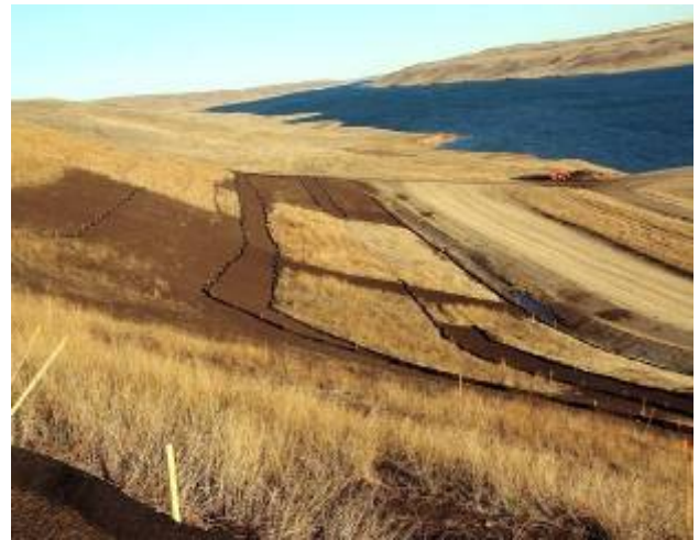
Completed compost berm and blanket (Nov 2008)
