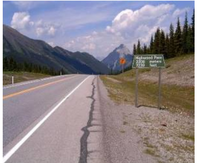
Highwood Pass on Highway 40
