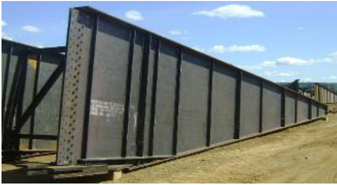
Temporary launching nose will be bolted to leading end of permanent girders to accommodate dead load deflection.
