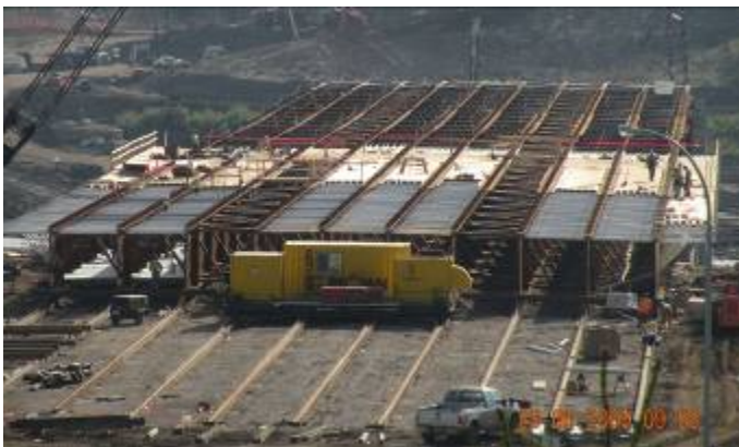
Girder segments pre-assembled adjacent to abutment and pushed incrementally across bridge piers
