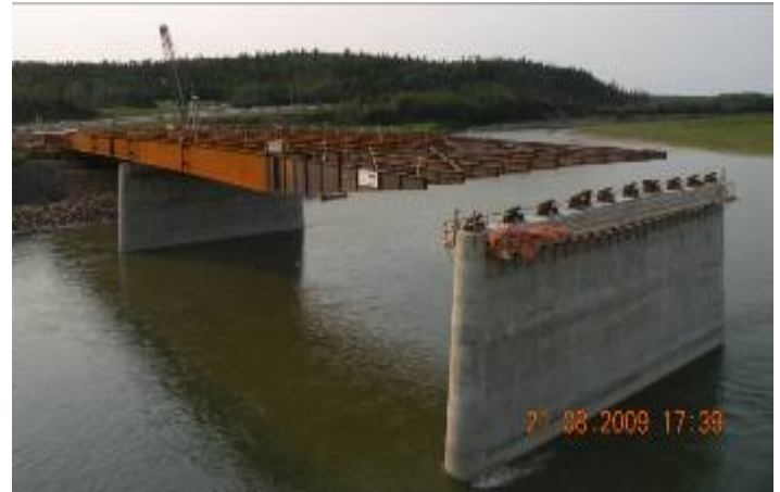
Launching in progress. Millions of pounds of structural steel pushed by customized equipment. During process, tapered launching nose touches down on top of landing pier rollers and lift permanent girders upward into position
