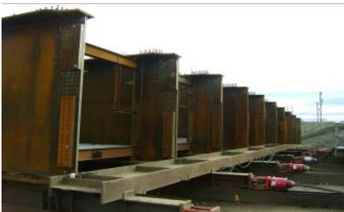
End of the girders at launching pad connected with tie beam. Strand jacks mounted at end of each of launching rails and operate with 4-18mm diameter strand.
