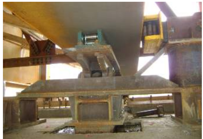
Vertical bearing rollers support each girder on its bottom flange, horizontal guide rollers provide alignment control.
