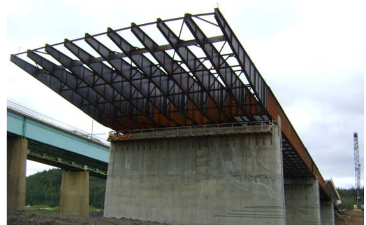
View of launching in progress.
