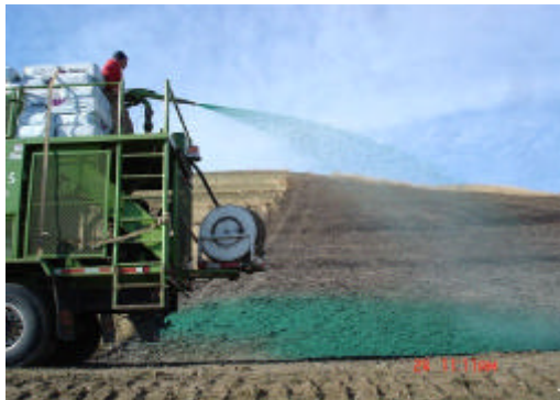
Application of standard hydro-seeding on buffers
