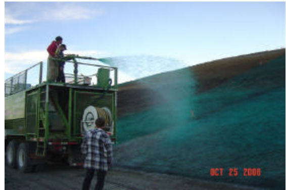
Application of Flexterra FGM
