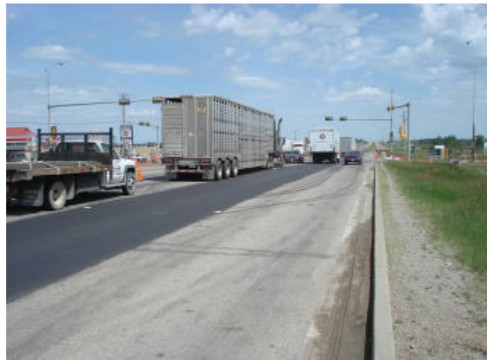
Photo 2 – Finished Product Hwy 1:12 EBOL at Lakeside Blvd.
