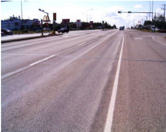
Photo 1 – Hwy 1:10 Severe Rutting
