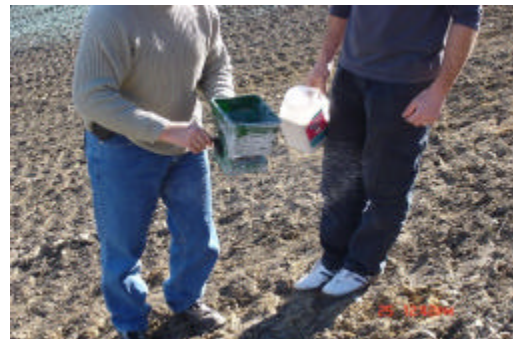
Application of Silt Stop
