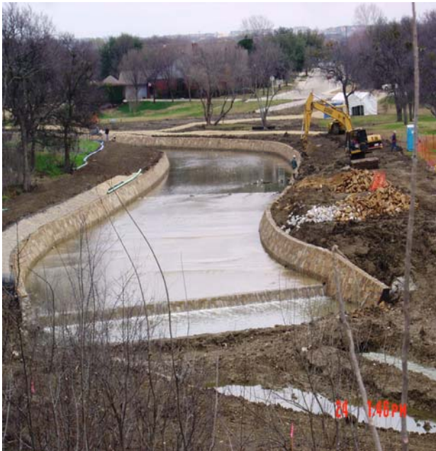
Furneaux Creek Channel Restoration
