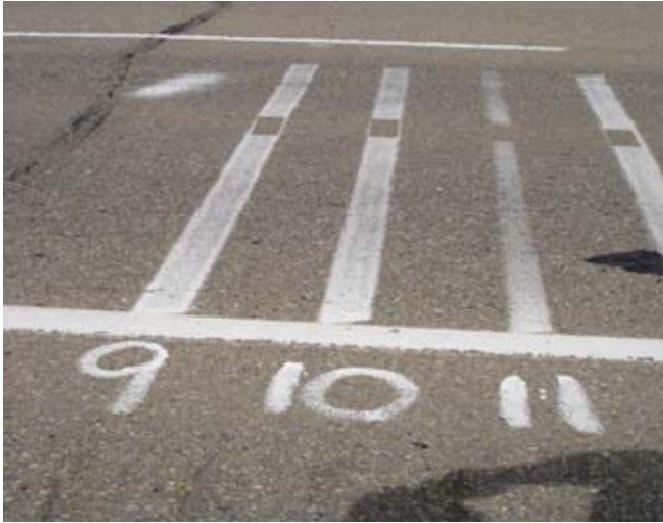
White paint, line #9 – 15mil, line #10 – 13mil and line #11 – 12mil The 12mil line (#11) is almost completely worn. The 13mil line (#10) is performing well.
