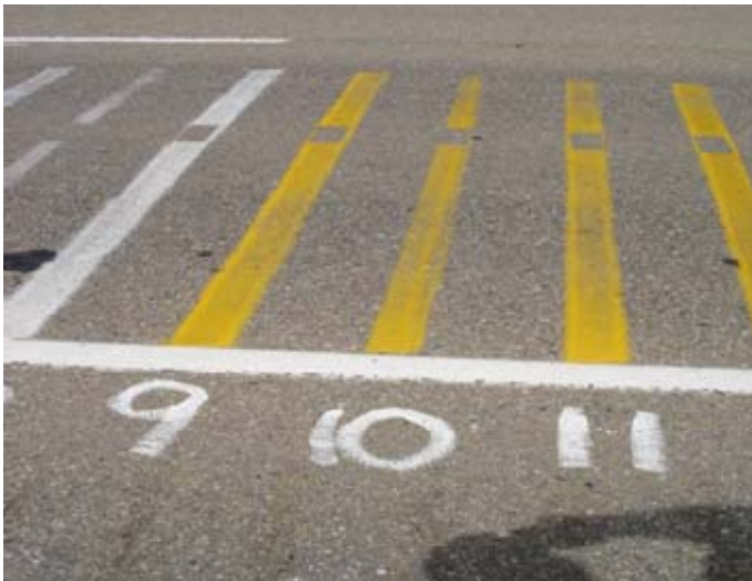
Yellow paint, line #9 – 15mil, line #10 – 12mil and line #11 – 13mil The 12mil line (#10) is almost transparent. The 13mil line (#11) is performing better.
