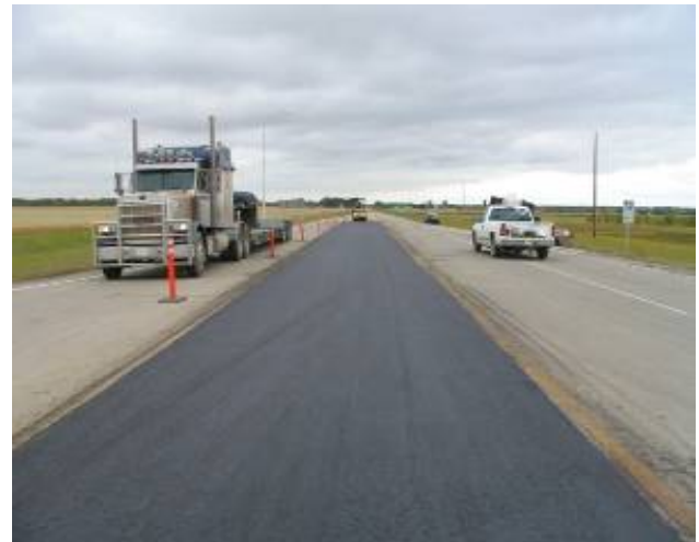
Photo 2 - Inlay of Hwy 37 at the Jct. of Hwy 44
