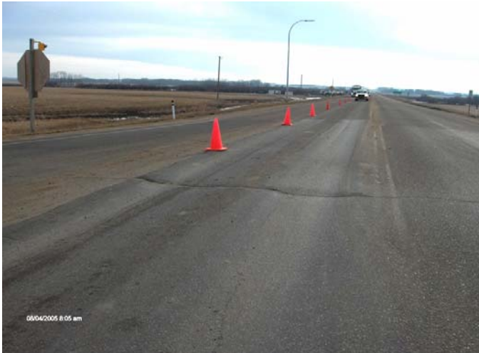
Photo 1 - Rutting at Jct. of Highway 37 and 44.
