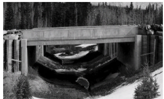
Three Sisters animal underpass
