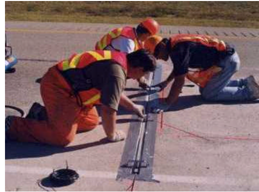
Installing Piezo Sensor into Slot Edson WIM Site 1999.09.16
