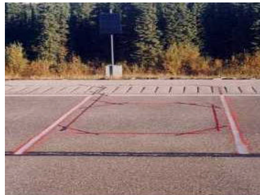
Completed Installation Edson WIM Site 1999.09.16
