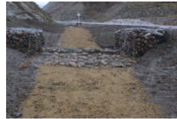
Geo Cell (brown gravel) channel
