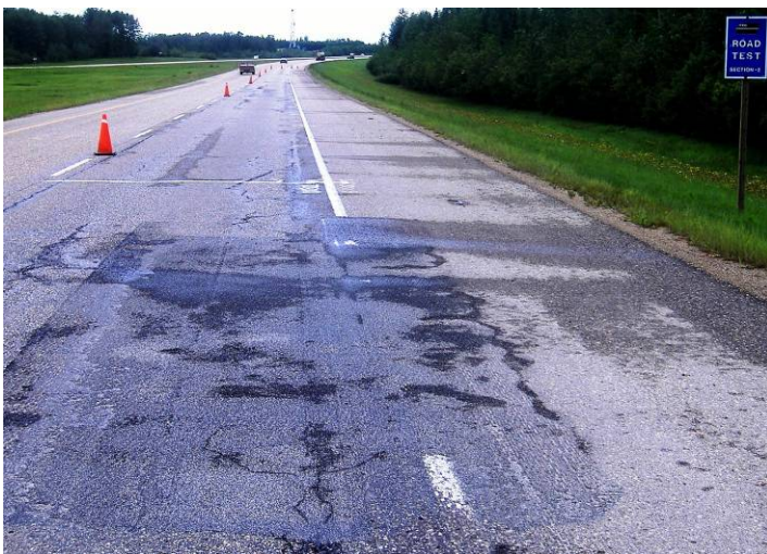
Photo 1. Blue Background Sign on Shoulder – SHRP Road Test
