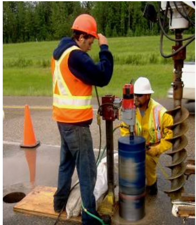
Photo 5 Coring 305mm diameter and Base Course Drill
