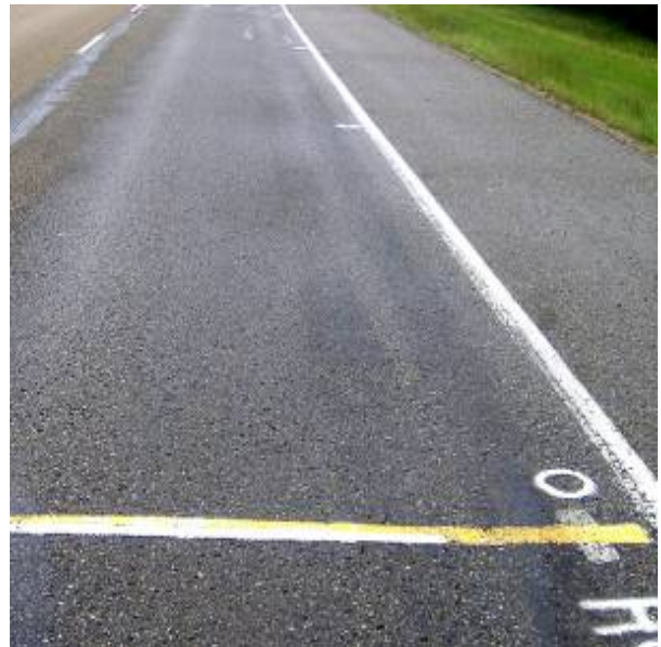
Photo 2 LTPP Section 04 127 mm overlay Hwy 16:06 June 2006
