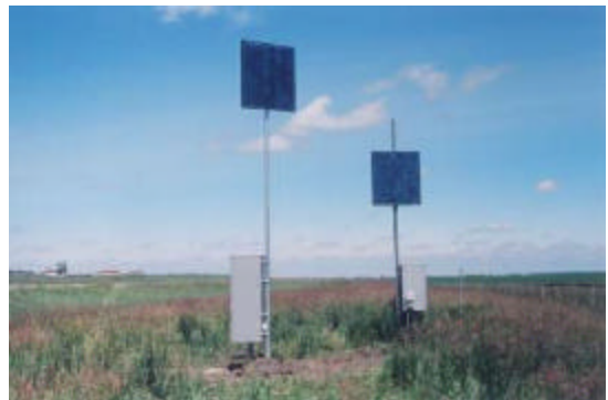
WIM Hwy 3:08 KM 13 4 Lane Instrument Cluster (left) Old cluster is on the right and will be recycled.
