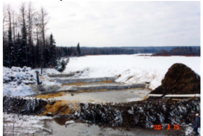
1-5 Silt retaining barrier/basin setup onsite to trap suspended material in water pumped out from pier excavation
