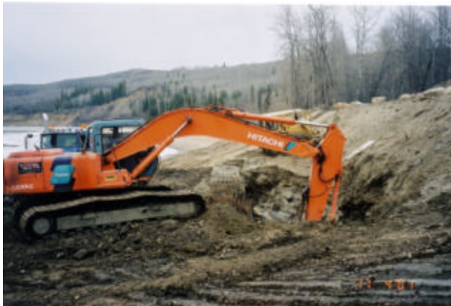
1-2 Pier excavation near the toe of headslope
