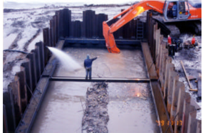
1-4 Pier excavation inside cofferdam - pumping water into cofferdam to equalize lateral pressure on walls
