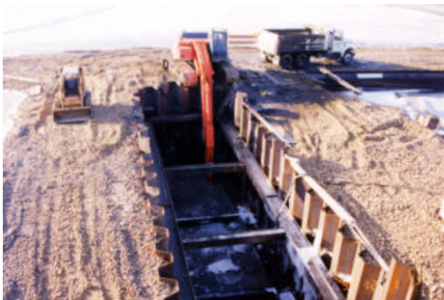
1-3 Pier excavation inside cofferdam in winter months
