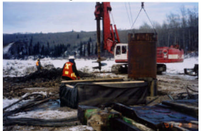
1-6 Silt trap setup onsite for filtering suspended material in water pumped out from drilled pile
