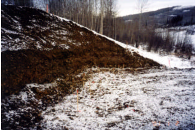
1-1 Abutment excavation near the top of headslope
