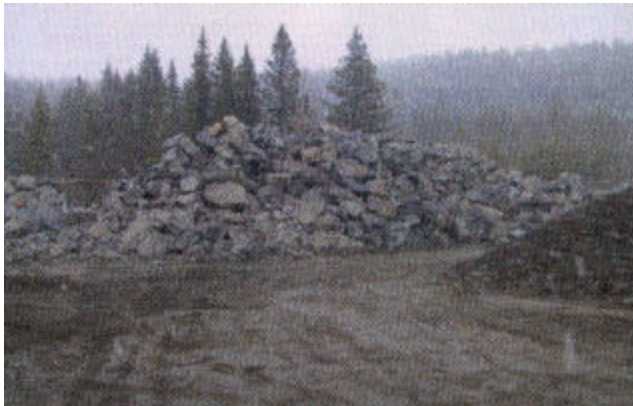
10-8 Heavy rock riprap stockpile
