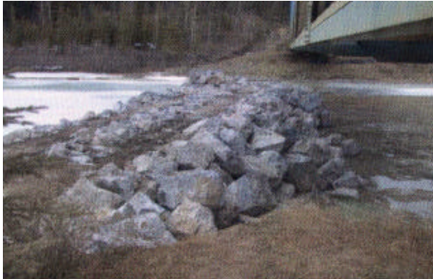
10-7 Placing heavy rock riprap
