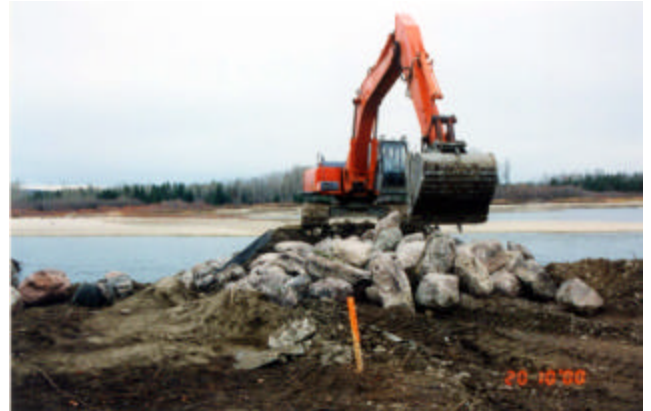
10-10 Placing heavy rock riprap
