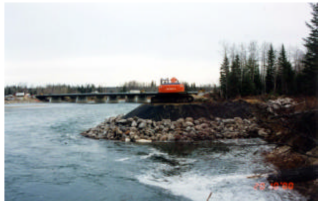
10-11 Placing heavy rock riprap on spur
