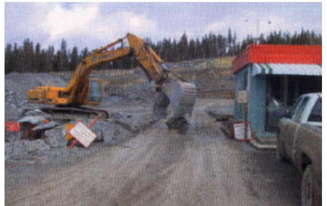
10-5 Weighing heavy rock riprap on the scale at the pit
