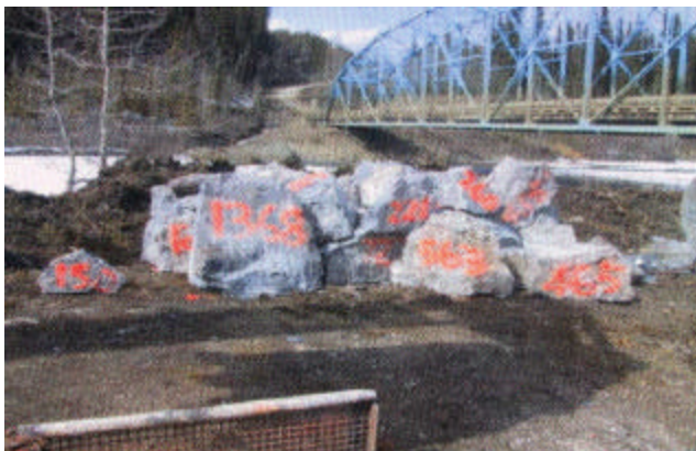
10-3 Heavy rock riprap sampled at site with weights painted on each rock
