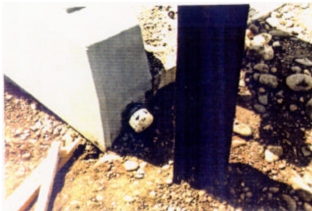
11-2 Service duct and void at end of curb
