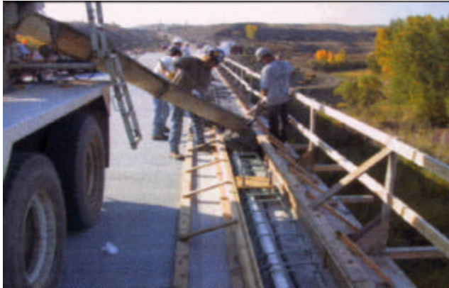
11-1 Service duct and void located in curb
