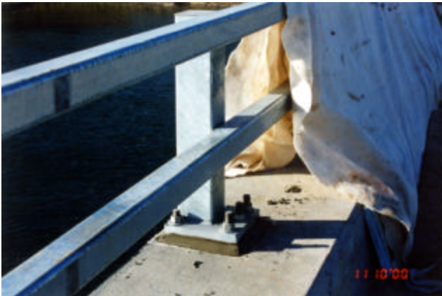
12-14 Typical completed bridgerail post grout pad
