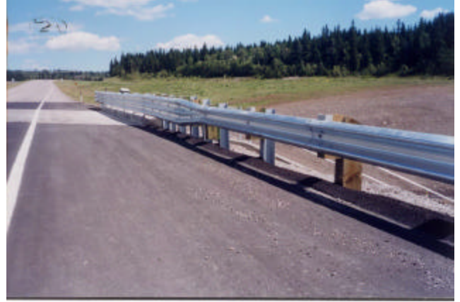
12-11 New Thriebeam bridgerail and approach transition
