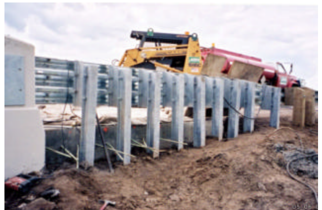
12-18 Thriebeam transition steel post spacing detail
