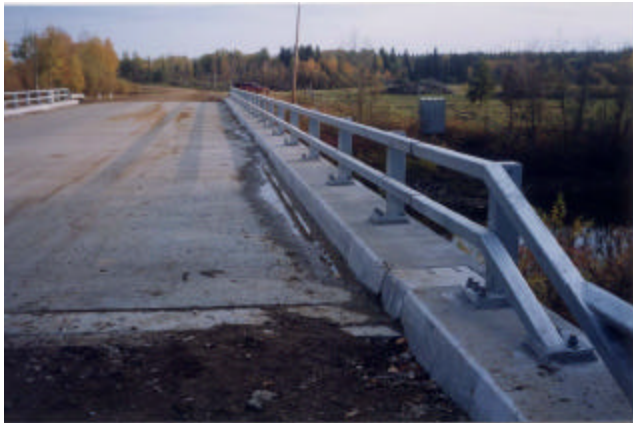
12-2 Old standard double tube bridgerail (1969-2000)
