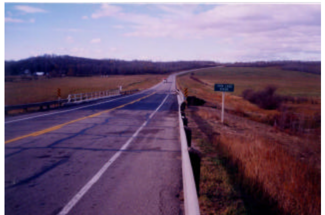
12-6 Re-aligning guardrail to shield projecting curb
