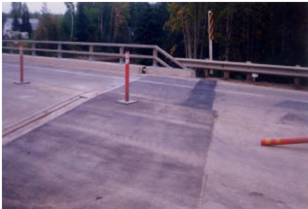
12-3 Old standard approach guardrail transition (1969-2000)
