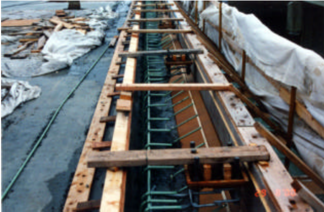
12-13 Typical deck curb formwork with bridgerail post anchor bolt assemblies installed
