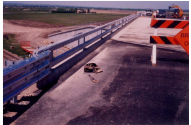
12-10 New standard bridgerail/Thriebeam connection
