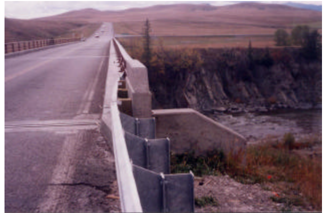
12-5 Re-aligning guardrail to shield bridgerail and curb end
