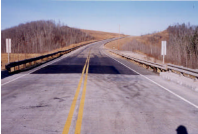
12-7 Old W-beam bridgerail with discontinuous approach guardrail
