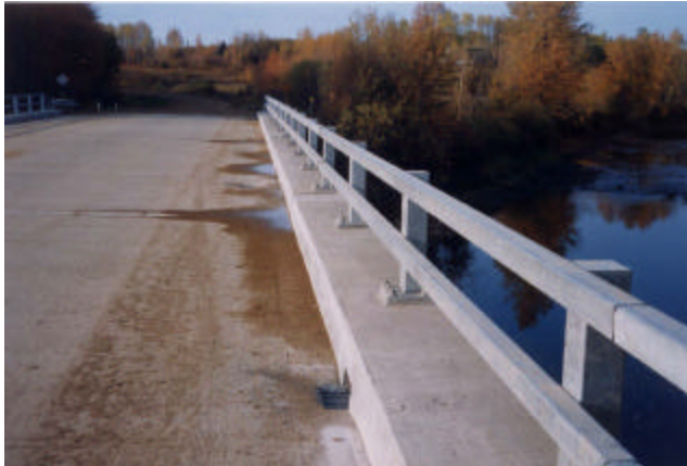
12-1 Old standard double tube bridgerail (1969-2000)
