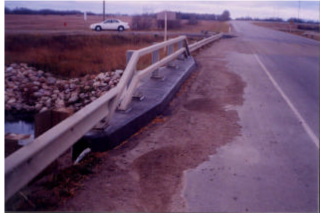
12-4 Curb projecting in front of bridgerail
