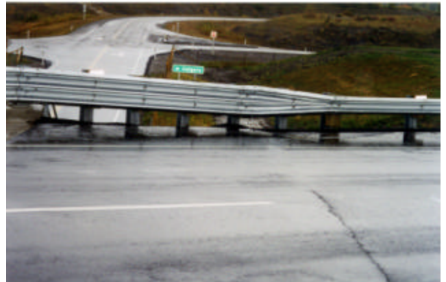
12-16 Approach Thriebeam to W-beam transition
