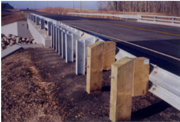
12-8 New Thriebeam transition to approach guardrail
