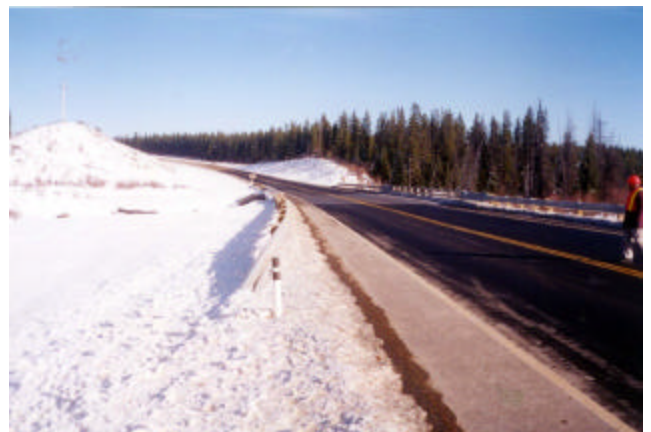
14-6 SW corner approach guardrail alignment suits situation
