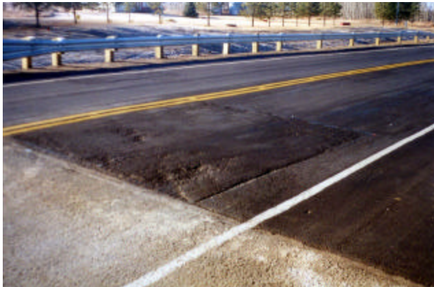
14-8 W-beam approach guardrail post spacing (1905 mm) closer to the bridge
