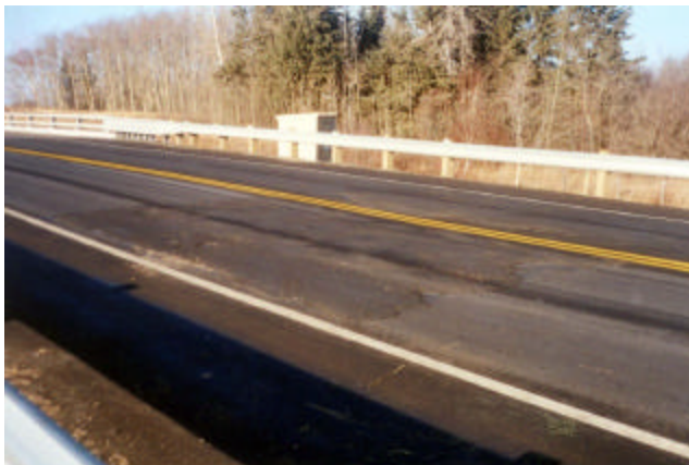
14-9 W-beam approach guardrail post spacing (3810 mm) farther away from the bridge
