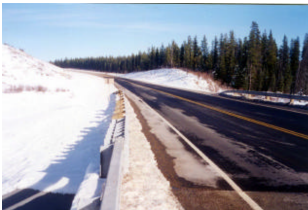
14-3 NW corner has been installed straight
