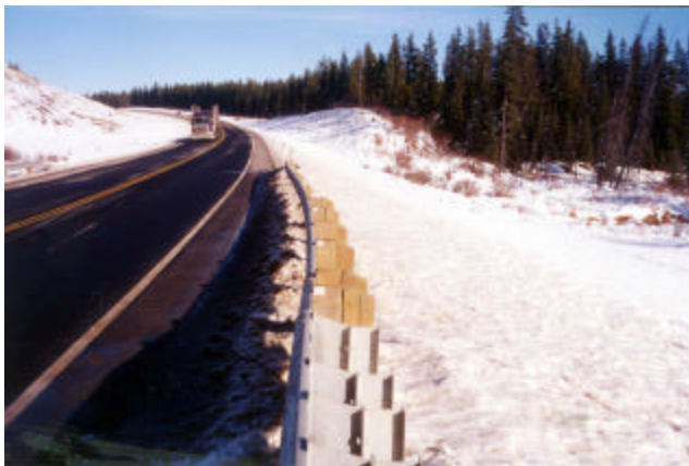
14-2 NE corner has been installed on curvature
