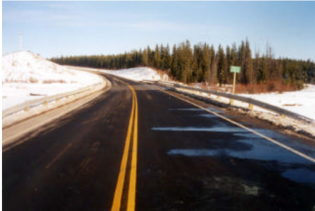
14-1 Approach guardrail to bridge
