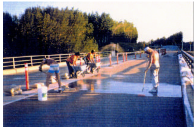
15-5 Applying polymer and seeding aggregates
