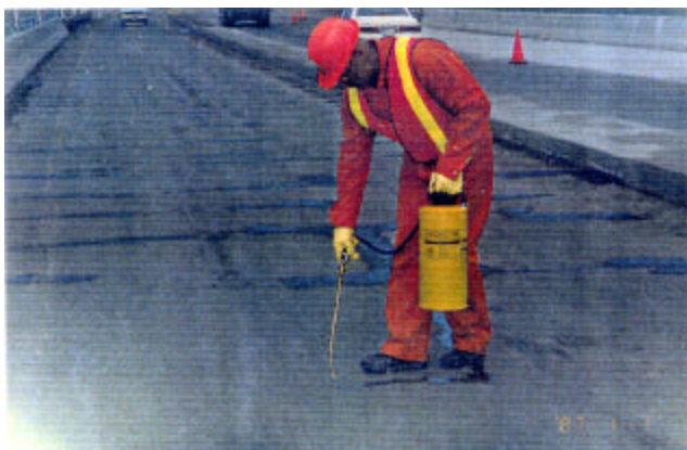
15-3 Sealing deck cracks
