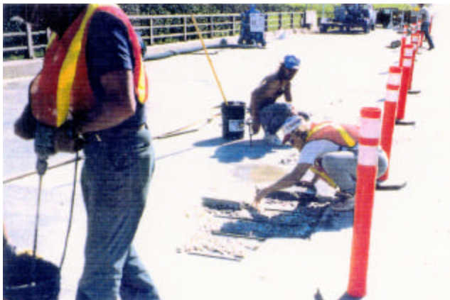
15-2 Partial depth repair
