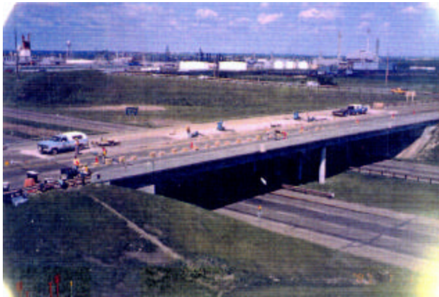
15-1 Deck surface preparation
