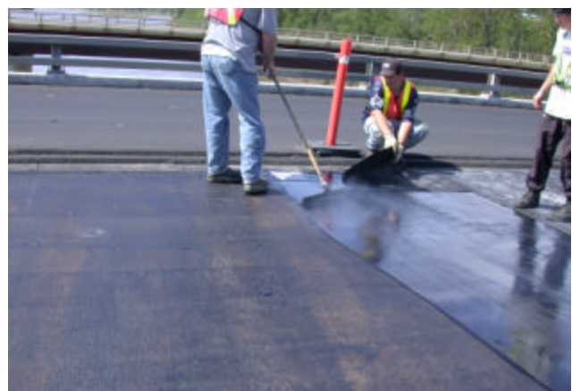
16-6 Applying hot waterproofing membrane and protection board
