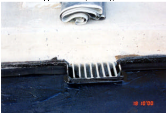
16-9 Wick drain running horizontally along curb into rectangular deck drain prior to placing of protection board
