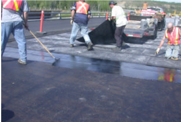
16-7 Placing protection board on top of hot-applied waterproofing membrane
