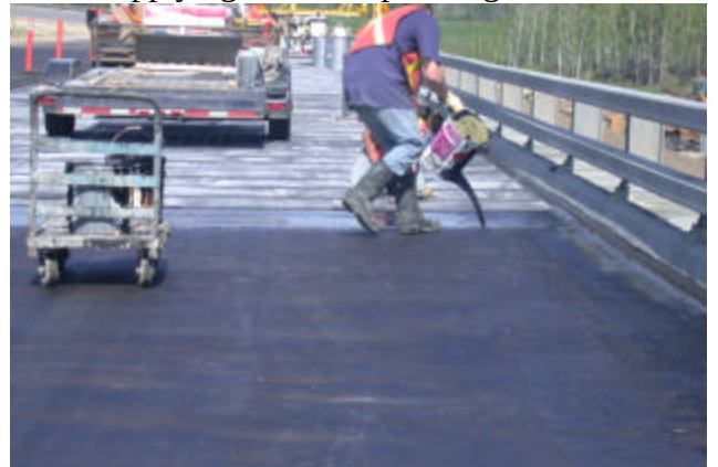
16-5 Applying hot waterproofing membrane
