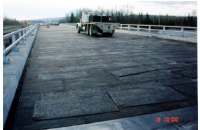
16-11 Waterproofing completed with wick drain running horizontally along curb
