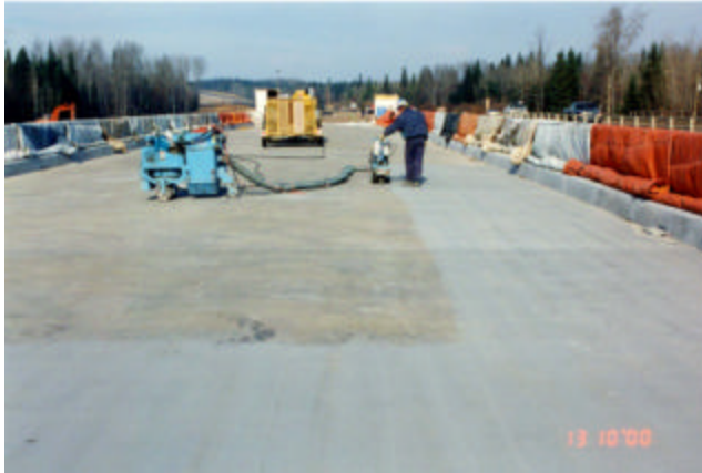
16-1 Surface preparation by shot-blasting
