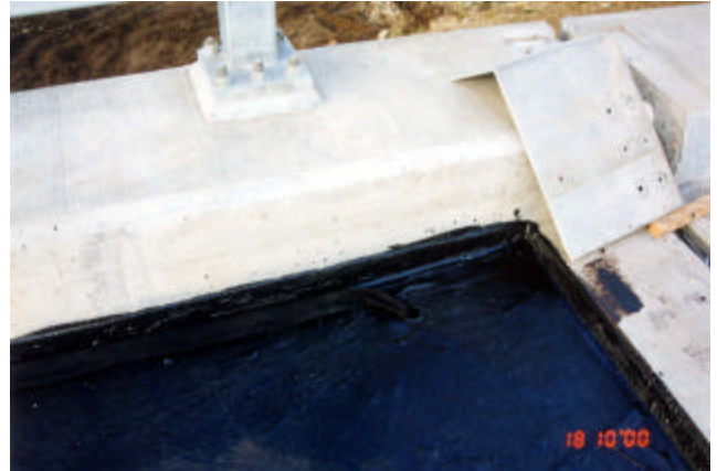
16-10 Wick drain running into weeping drainpipe at abutment
