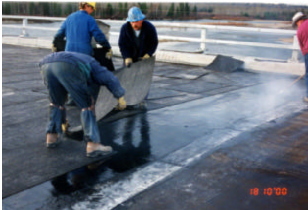
16-8 Placing 300 mm wide butyl rubber membrane over construction joint prior to hot-applied waterproofing membrane
