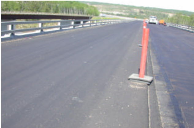
16-2 Apply tack coat to bridge deck prior to waterproofing
