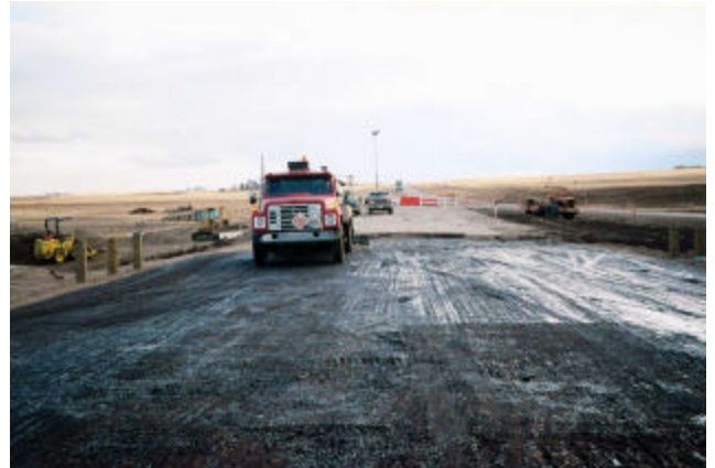
17-4 Applying tack coat
