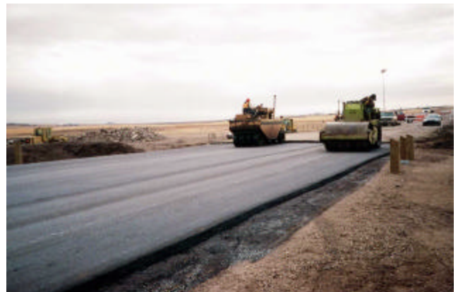
17-6 Compacting ACP with steel drum roller and wobbly
