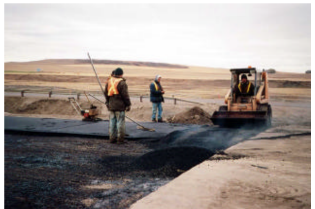
17-5 Spreading ACP with Bobcat along sawcut of existing roadway ACP
