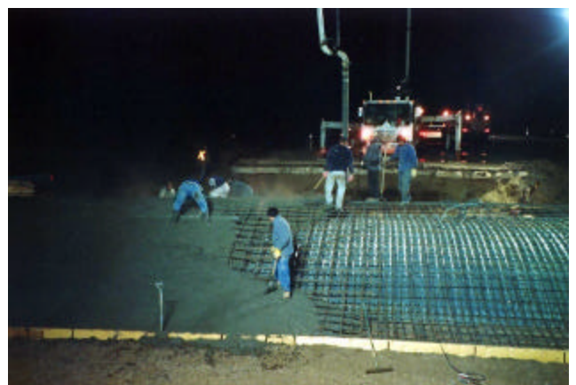
18-23 Night placement of concrete
