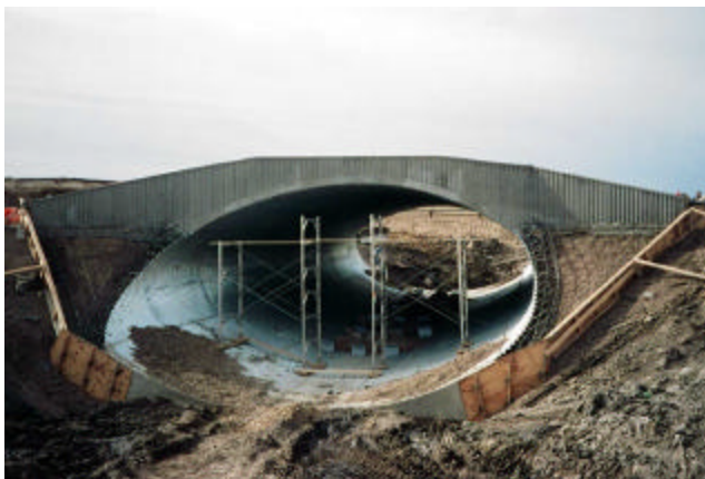
18-21 Formwork for concrete slope protection
