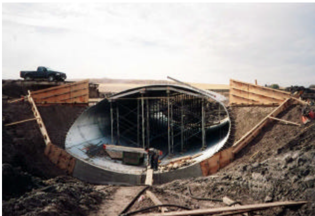
18-20 Shoring in place for concrete placement
