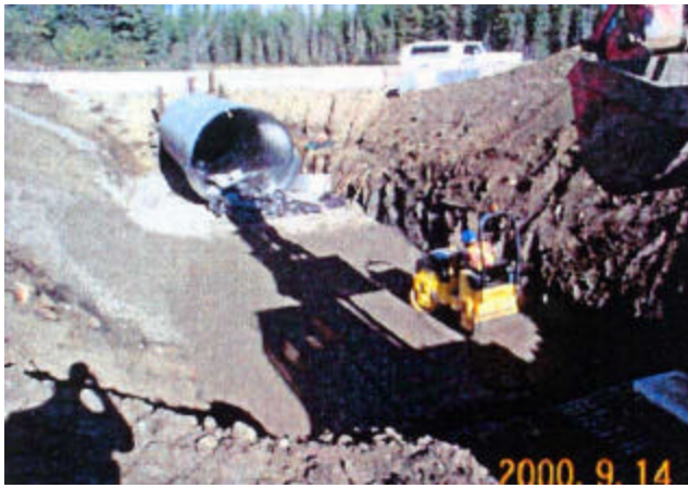
18-2 Installation of CSP
