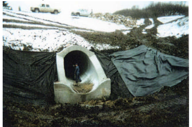
18-12 Completing upstream end of SPCSP
