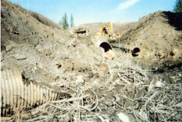
18-7 Removal of the existing culvert and structural excavation
