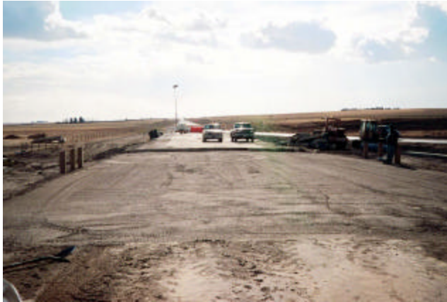
18-25 Backfill and granular base course completed over culvert
