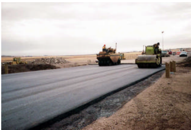
18-27 Paving over culvert
