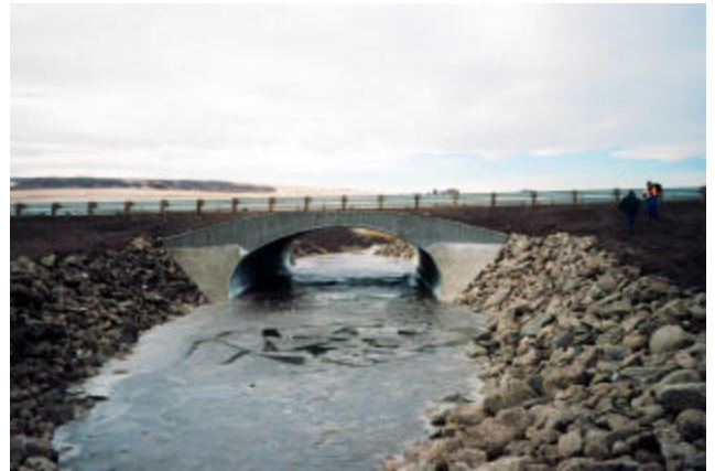
18-28 Downstream end of completed culvert
