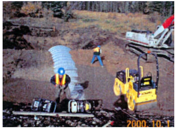
18-5 Backfill near the top
