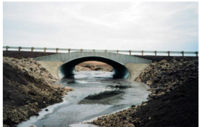
18-29 Upstream end of completed culvert
