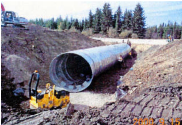
18-3 Assembling CSP with fish baffles pre-assembled in the shop
