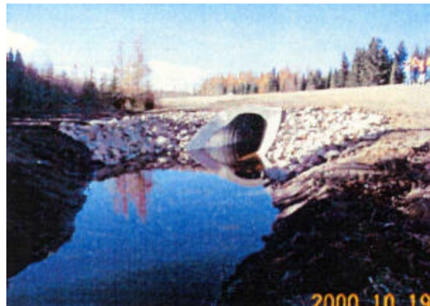
18-6 Completed upstream end of CSP
