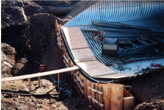
18-19 Cut-off wall ready for concrete placement
