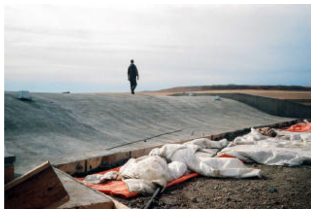
18-24 Concrete slab complete
