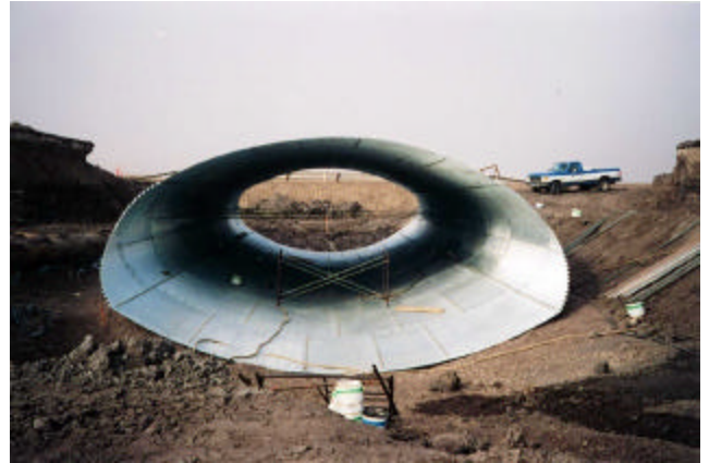
18-16 Assembling horizontal ellipse SPCSP
