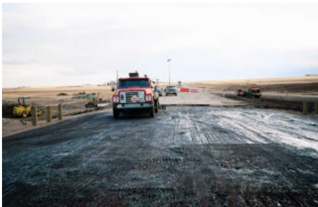
18-26 Applying tack coat to granular base course surface prior to paving
