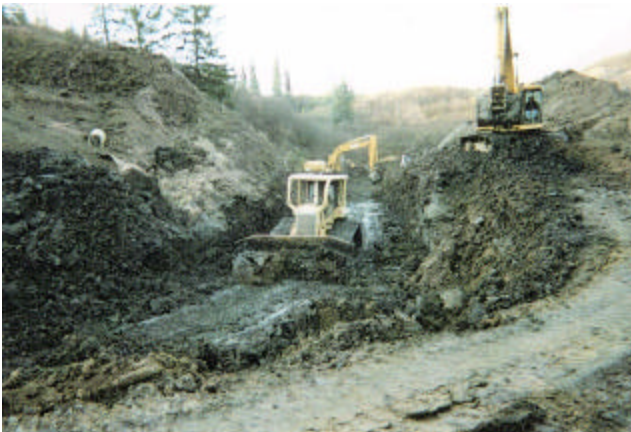
18-8 Culvert bed excavation - 0.6 m undercut
