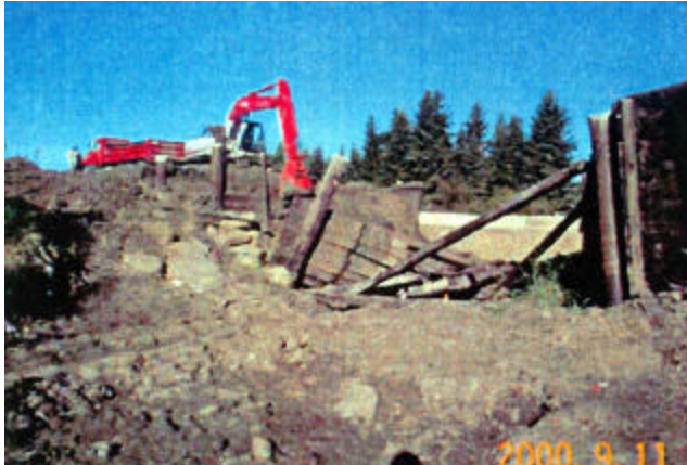
18-1 Structural excavation and removal of the existing bridge structure
