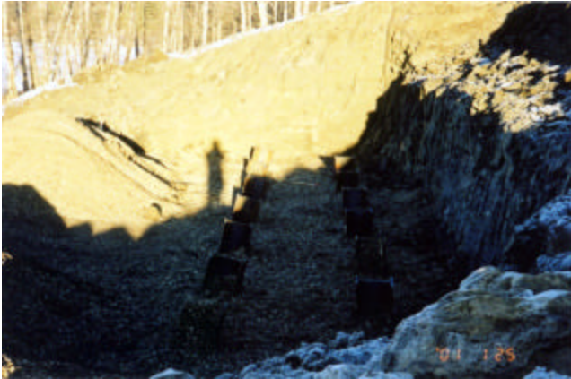
2-1 Compacted granular backfill under abutment seat
