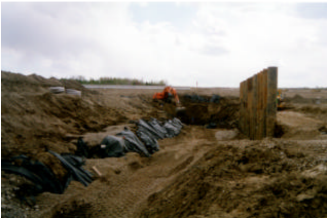
2-2 Soft yielding material replaced with competent granular backfill
