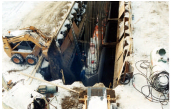
2-5 Placing unfrozen backfill into pier excavation with a bobcat
