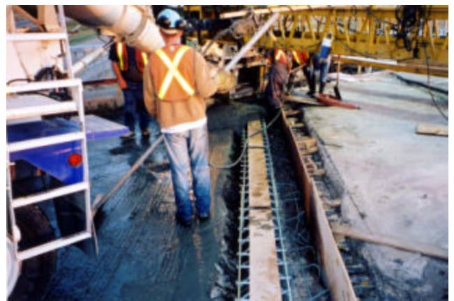
20-17 Placing abutment deck joint concrete monolithic with deck overlay concrete
