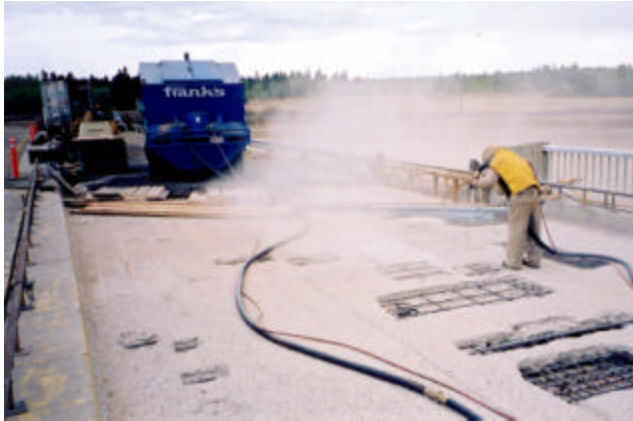
20-13 Surface preparation consists of sandblasting deck concrete
