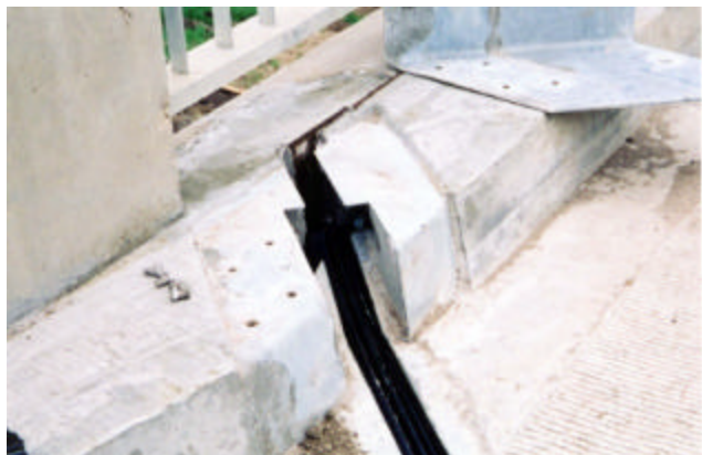
20-21 Abutment joint deck detail at curb
