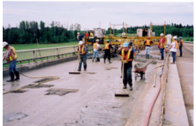
20-16 Grout slurry being applied to deck prior to concrete placement
