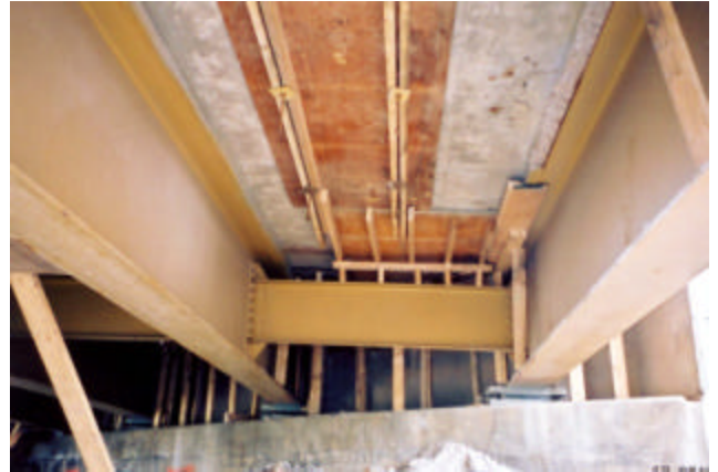
20-4 Typical forming of full depth repair at the underside of deck.
