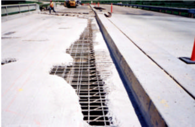
20-7 Substantial full depth repair area.
