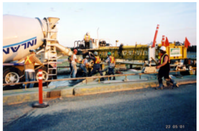
20-12 Placing and finishing deck overlay concrete
