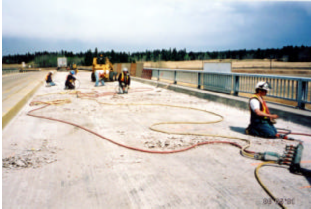
20-1 Chipping partial and/or full depth repair areas on bridge deck.
