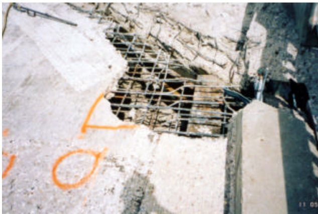
20-2 Full depth repair area
