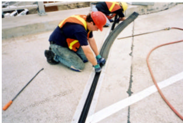
20-20 Installation of abutment joint compression seal
