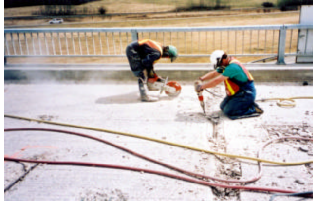
20-10 Sawcutting and chipping deck concrete for pier deck joint replacement
