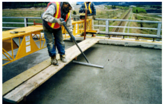
20-29 Surface texture consists of transverse grooving
