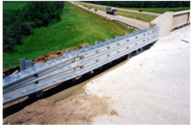
20-23 Approach guardrail upgrading - Retrofit thrie-beam transition
