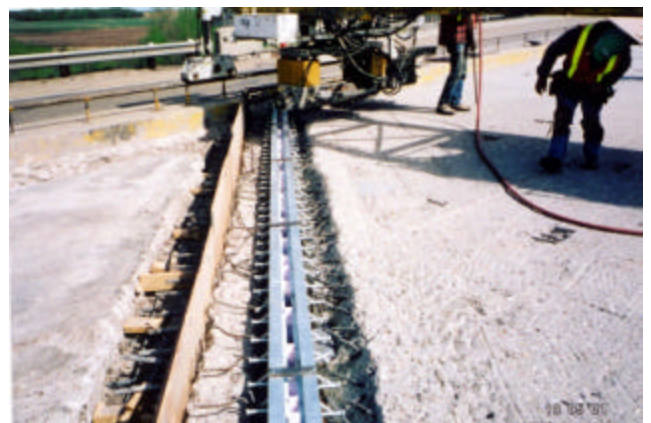
20-11 Abutment deck joint in place and ready for concrete pour
