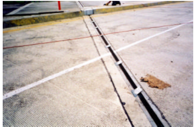
20-22 Abutment deck joint complete
