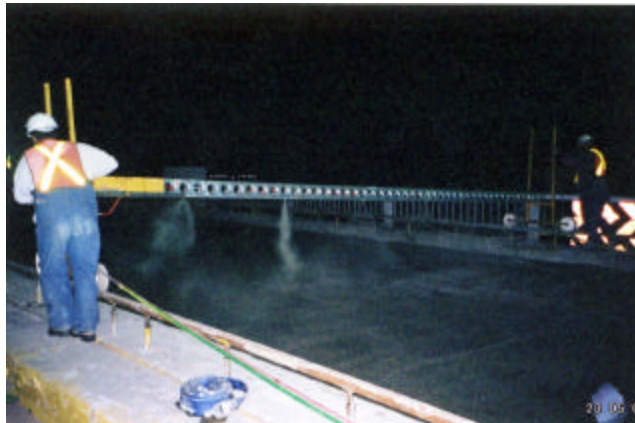
20-19 Fog misting overlay concrete
