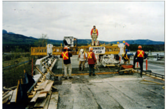
20-28 Placing and finishing deck overlay concrete with screeding machine
