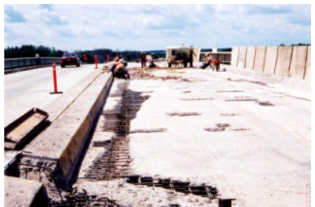
20-6 Substantial full depth repair area.
