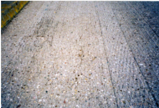
20-14 Typical sandblasted deck surface
