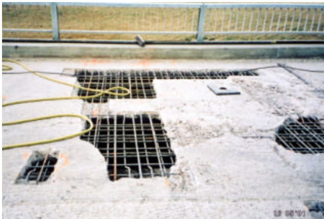
20-3 Full depth repair areas chipped out.
