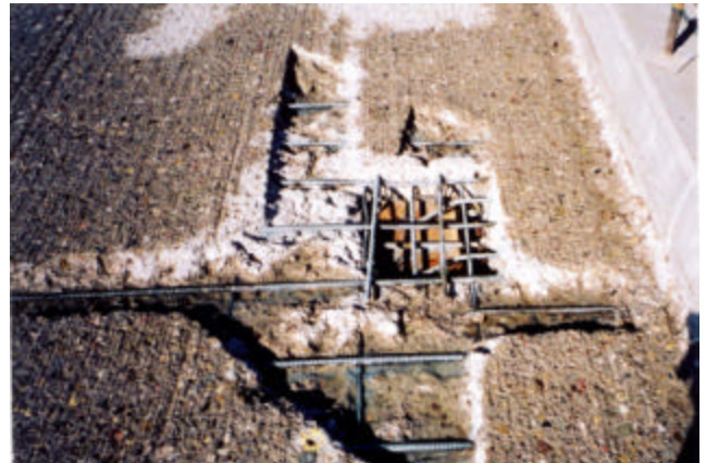
20-5 Full depth and partial depth repair in one area.
