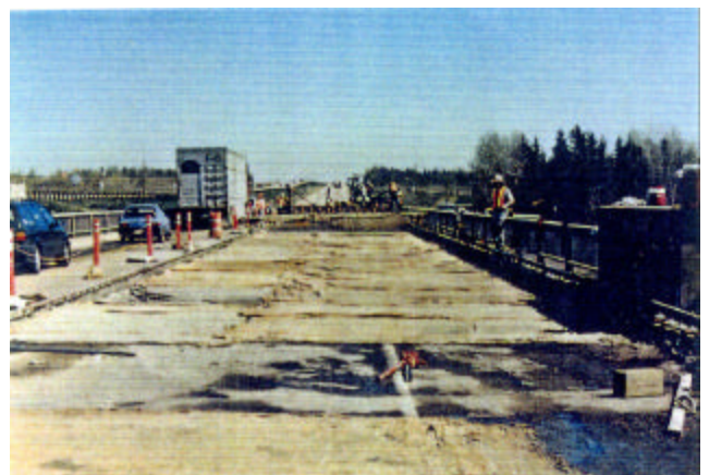
20-30 Wet curing of deck overlay concrete
