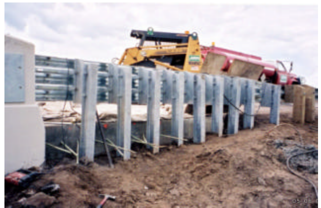
20-24 Retrofit thrie-beam transition post detail
