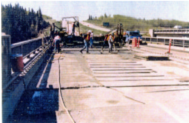
20-26 Applying slurry grout in front of finishing machine
