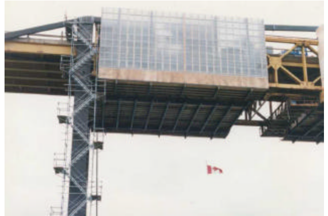
22-32 Staircase access erected inside tube and clamp scaffolding
