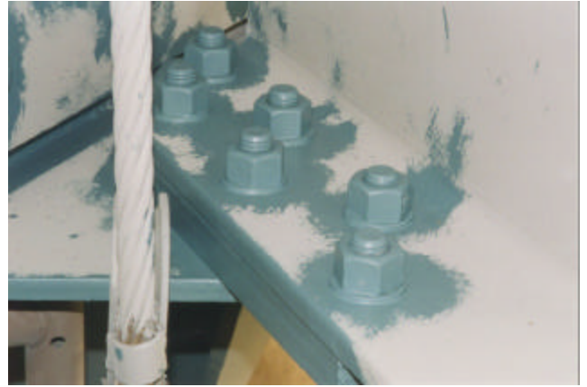
22-54 Prime coat striping prior to prime coating
