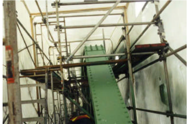
22-11 Inside of shrink-wrap containment structure
