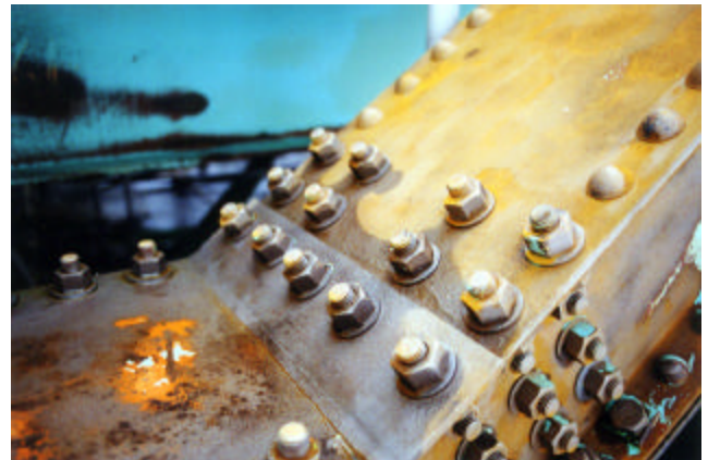
22-6 Check concentration of chloride after washing
