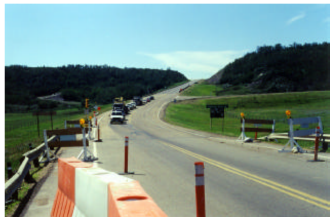
22-16 Traffic is stopped for the dismantling of scaffolding
