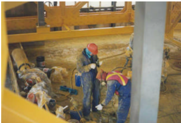
22-52 Painter setting up inside paint platform
