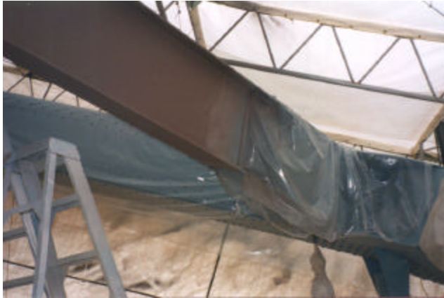
22-57 Prime coat is gray, intermediate coat is blue or brown
