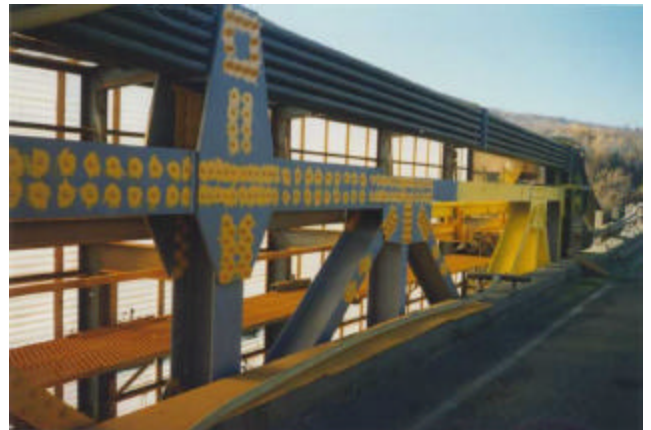
22-56 Top coat striping prior to top coating
