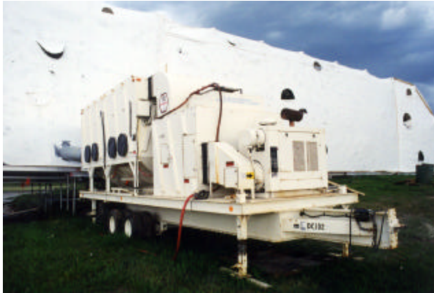
22-7 Dust collection unit parked beside shrink-wrap containment structure
