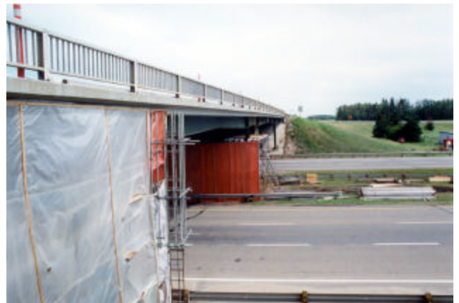
22-22 Clear tarp, tube and clamp scaffolding containment structure
