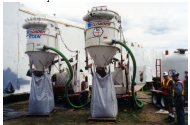
22-5 Sandblasting spoil vacuum recovery units
