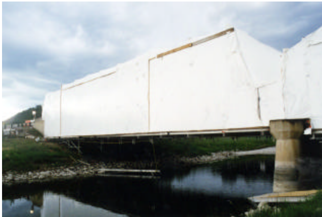
22-8 Shrink-wrap containment structure
