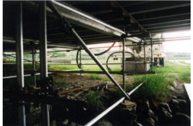
22-10 Tube and clamp scaffold platform on headslope
