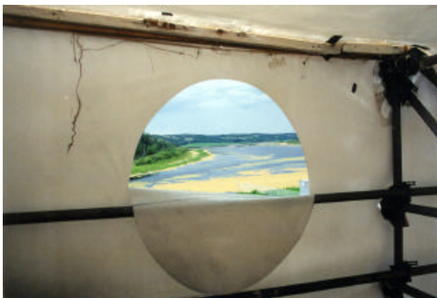
22-9 Shrink-wrap plastic opening for fresh air circulation
