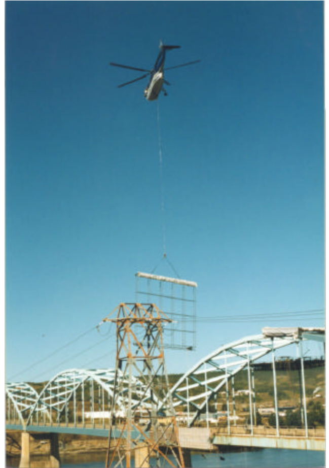
22-37 Scaffold erection by helicopter
