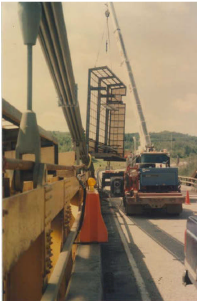
22-31 Scaffold erection
