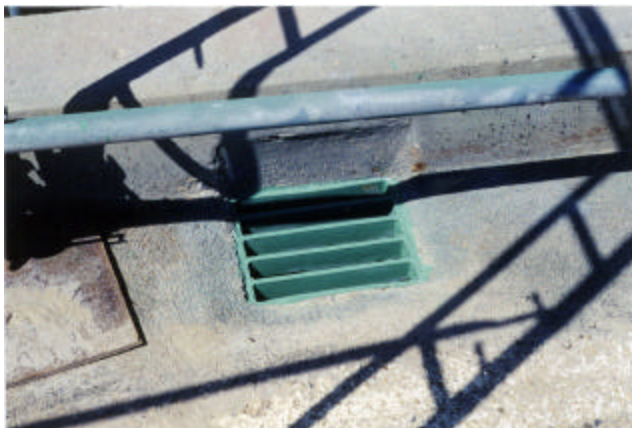
22-20 Conscientious Contractor sandblasted and painted deck drain
