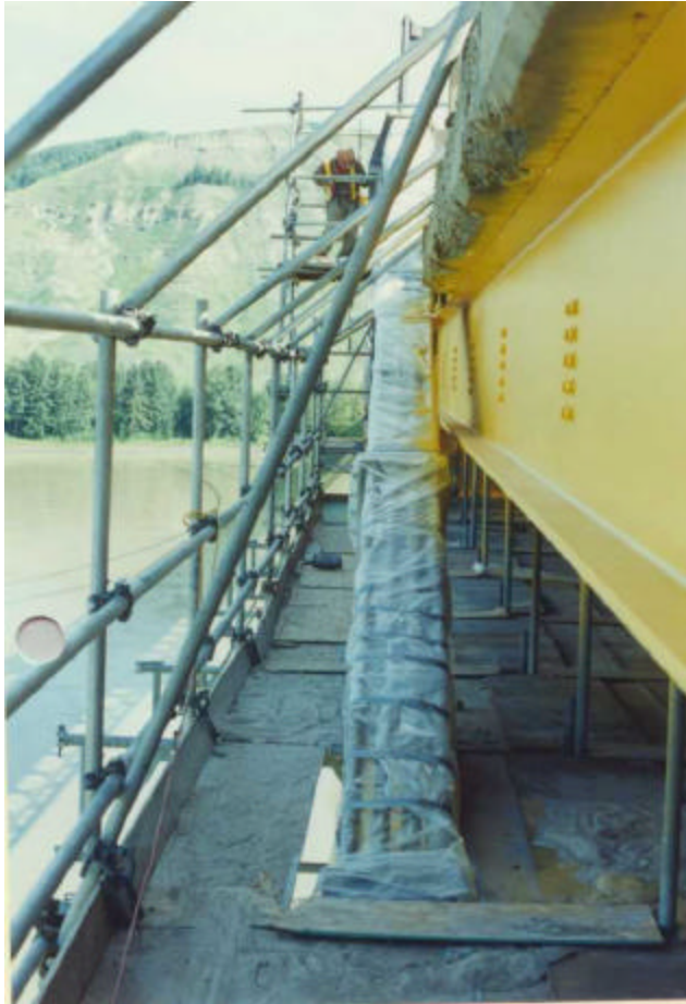
22-35 Tube and clamp scaffolding at approach spans
