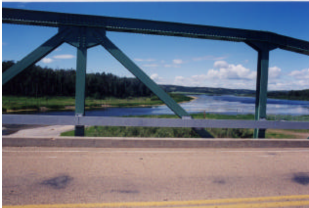
22-19 Galvanized bridgerail installed on brackets separated by neoprene gaskets
