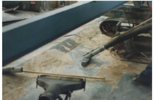
22-48 Vacuuming sandblast spoil from platform floor
