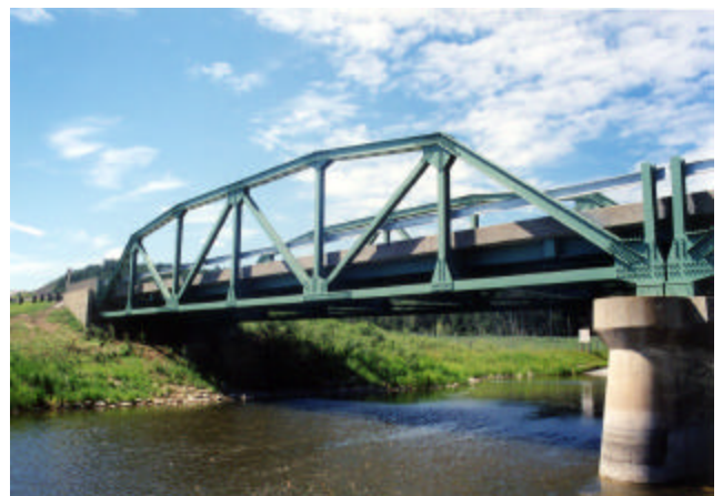
22-17 Profile view of freshly painted pony truss bridge
