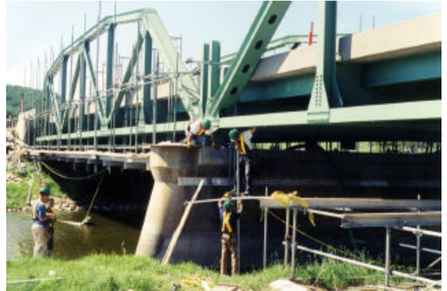
22-15 Dismantle tube and clamp scaffolding
