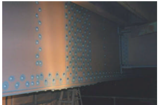
22-55 Intermediate coat striping prior to intermediate coating
