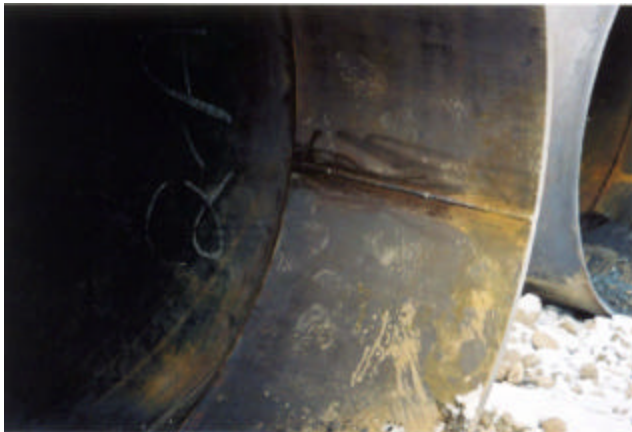
3-28 Pipe pile with tip reinforced
