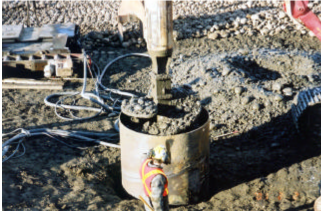
3-33 Material inside pipe pile being drilled out with an auger rig attachment
