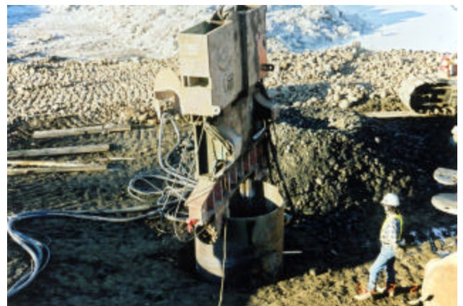
3-31 Advancing pipe pile with vibro hammer
