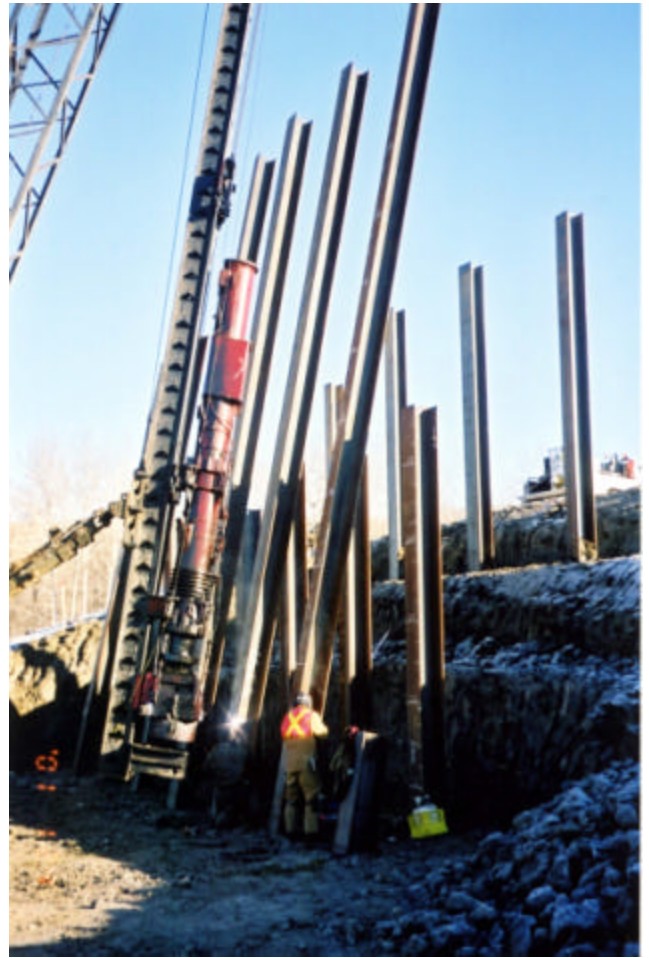
3-8 Delmag D30-32 diesel hammer driving H-pile to final set
