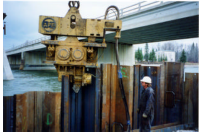
3-2 Advancing sheet piles with vibro hammer
