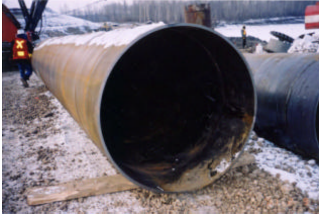
3-27 Pipe pile caissons
