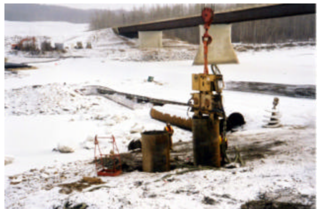
3-4 Advancing pier pipe pile caissons
