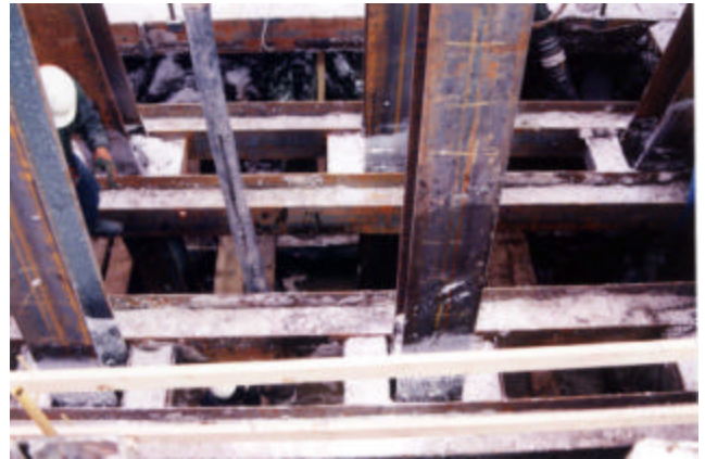
3-19 Pile driving frame at pier
