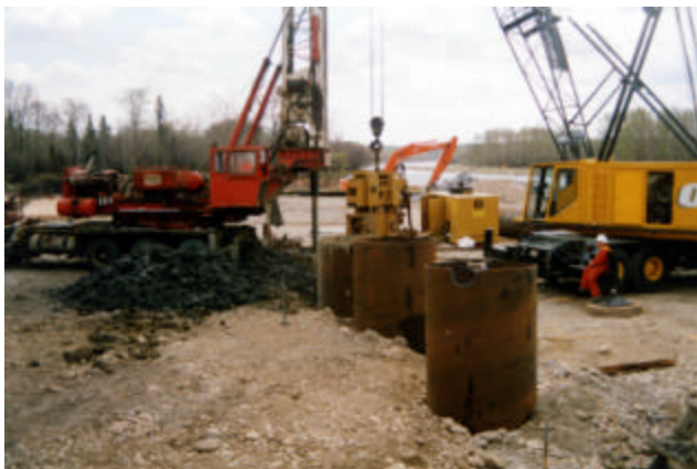
3-29 Pre-drilling for pile installation
