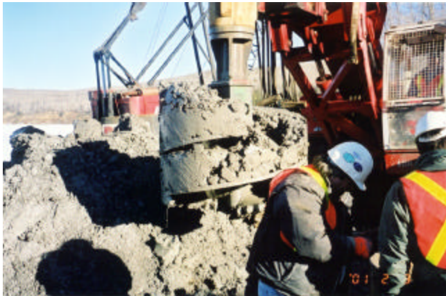
3-34 Examining tailings to see whether suitable bearing layer has been reached
