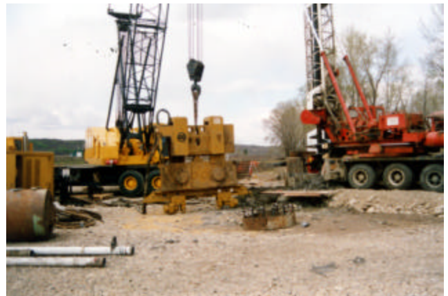
3-3 Vibratory Pile Driver for advancing pipe piles
