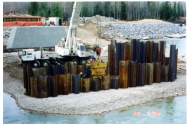
3-15 Subsequent piles advanced the same amount
