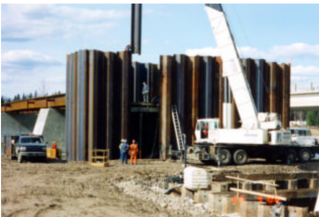
3-12 Thread sheet piles prior to driving
