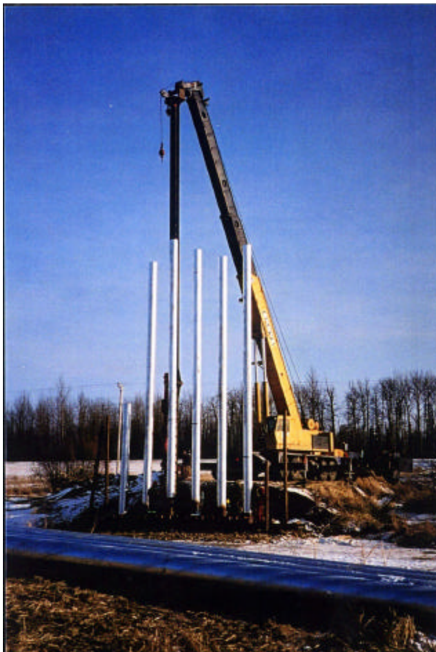
3-23 Galvanized pipe sections spliced onto plain pipe sections
