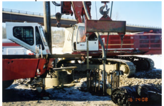
3-38 Pouring pile concrete after reinforcement has been properly placed
