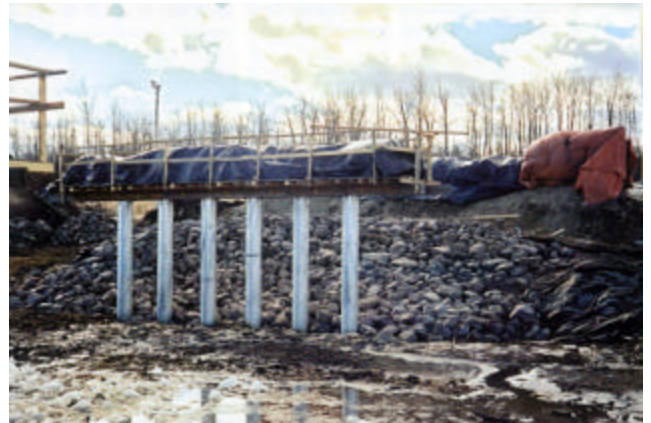
3-24 Galvanized pipe piles
