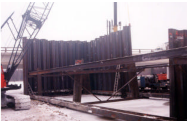
3-11 Setting up sheet piles
