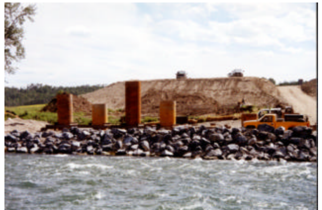
3-25 Pipe piles at pier
