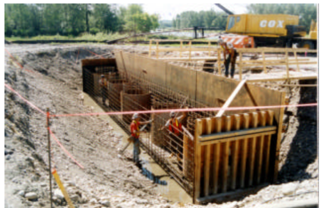
3-26 Pipe piles at abutment
