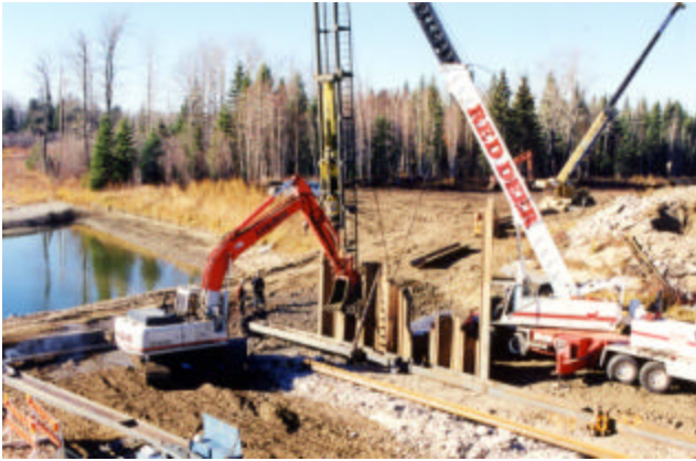
3-5 Birmingham B-3505 diesel hammer driving sheet piles
