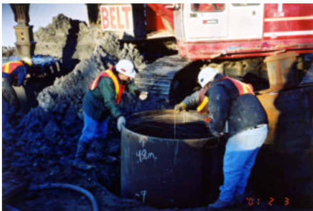
3-35 Checking pile tip elevation
