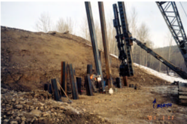
3-7 Delmag D19-32 diesel hammer driving first length of H-Piles at abutment
