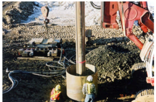
3-32 Removing material from inside pipe pile with drill rig
