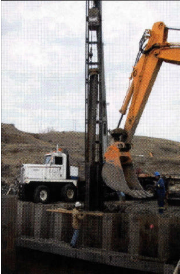
3-1 Drop hammer driving sheet piles
