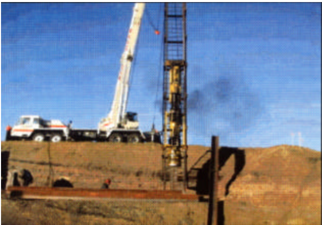
3-6 Birmingham B-4505 diesel hammer driving H-piles
