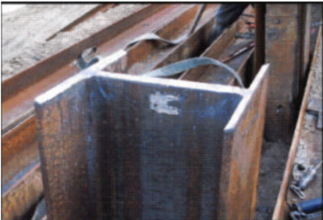
3-17 Field splice preparation
