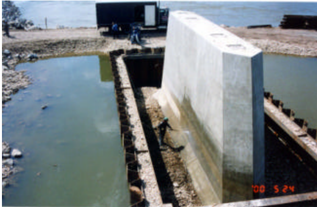
4-19 Sealer being applied to pier shaft after surface preparation
