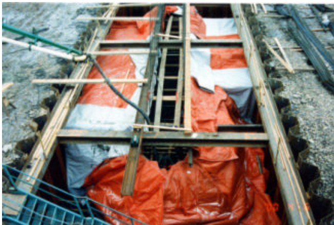
4-15 Placing pier footing concrete
