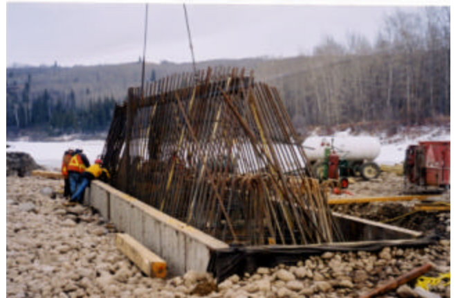
4-5 Pier footing (EFCO) form insulated with Styrofoam
