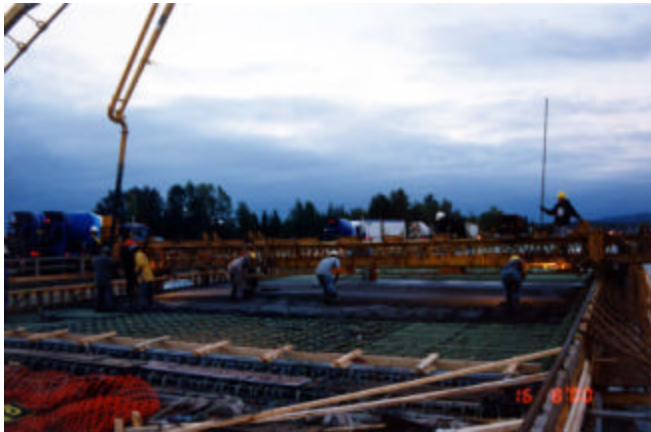
4-20 Deck pour at dusk when cooler temperature and no wind
