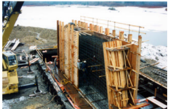
4-4 Pier shaft formwork
