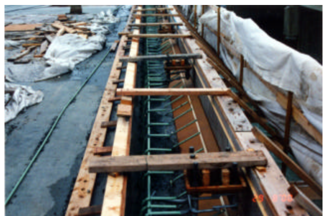
4-12 Deck curb form with bridgerail post anchor bolt assemblies installed
