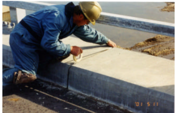
4-29 Masking tape used at bottom of reglet to debond caulking.
