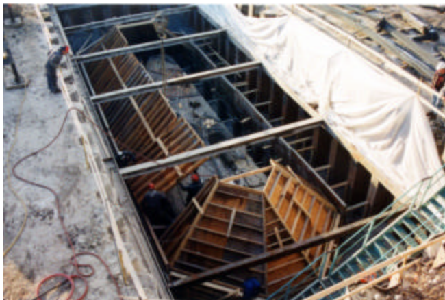
4-3 Pier footing formwork
