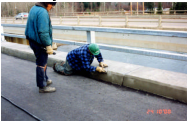
4-27 Using a carborundum stone to produce smooth and closed surface
