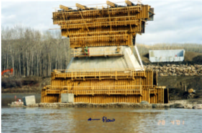
4-7 Upper pier shaft (EFCO) forms
