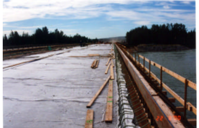
4-22 Wet curing for deck concrete for a minimum period of 7 days
