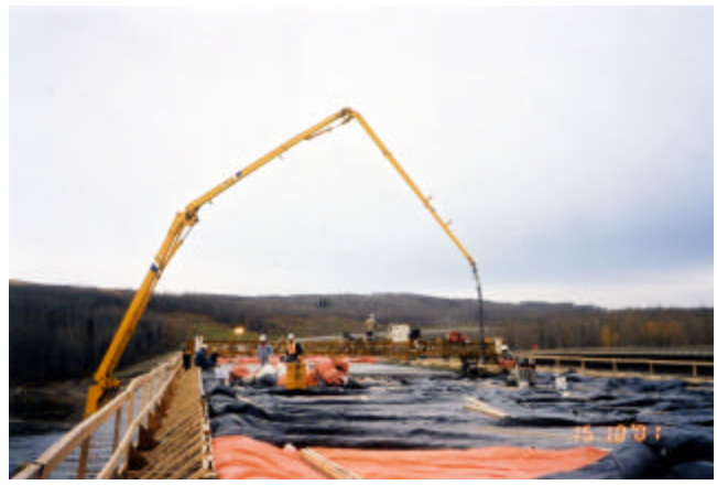
4-17 Placing and curing deck concrete under adverse weather conditions
