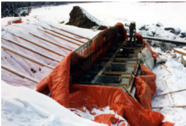
4-14 Cold weather concreting at abutment
