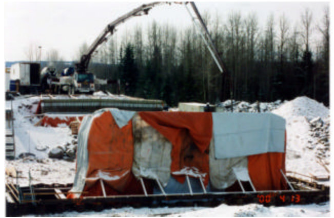
4-16 Placing pier shaft concrete in cold weather conditions
