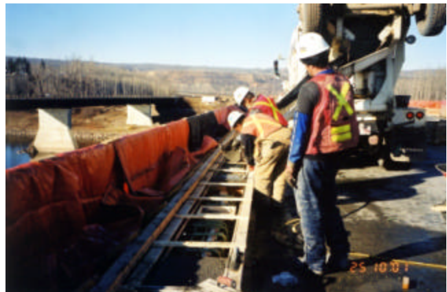
4-18 Placing and finishing curb concrete in alternate 3m long sections
