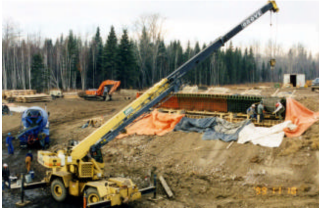
4-13 Placing abutment seat concrete with crane and hopper
