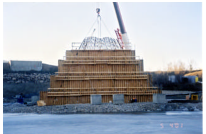
4-6 Lower pier shaft (EFCO) formwork
