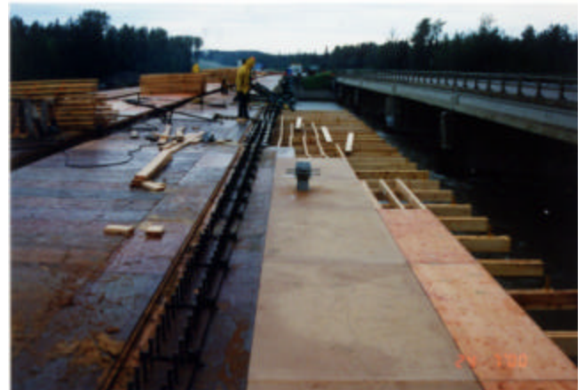
4-11 Deck soffit forms
