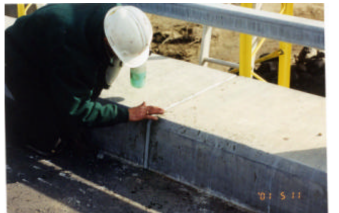
4-30 Curb construction joint being caulked
