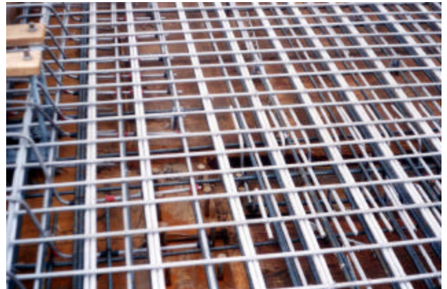
5-10 Stainless steel reinforcement detail over pier
