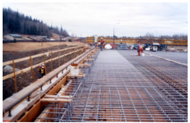
5-12 Curb and deck stainless steel reinforcement details
