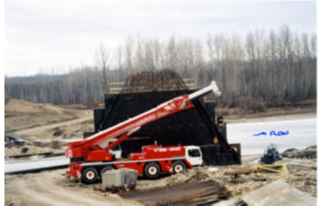
5-4 Lower pier shaft - Plain steel reinforcement
