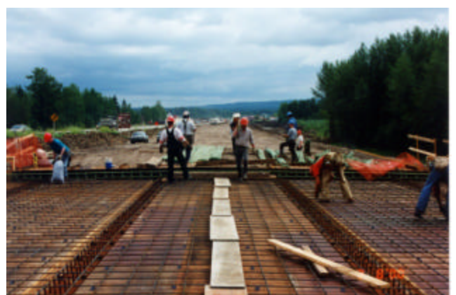
5-6 Bottom deck plain steel reinforcement
