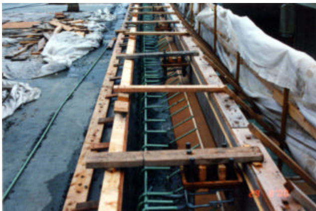
5-9 Epoxy coated reinforcing for curb
