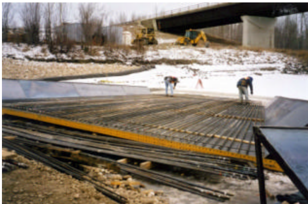
5-3 Pre-tying lower pier shaft steel reinforcement on EFCO form
