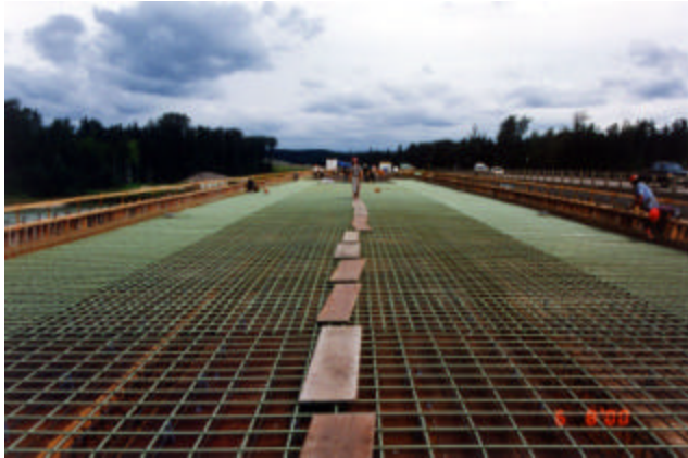
5-7 Epoxy coated reinforcement for top layer of deck slab
