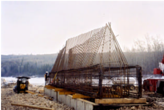
5-2 Pier footing plain steel reinforcement
