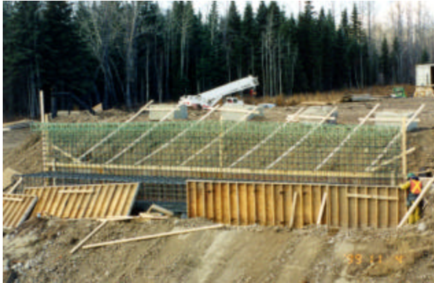
5-1 Top portion of abutment is epoxy-coated reinforcement
