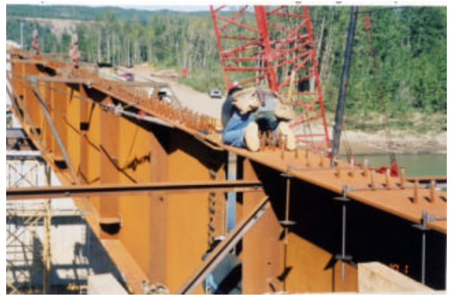
6-24 Splice connection in the air
