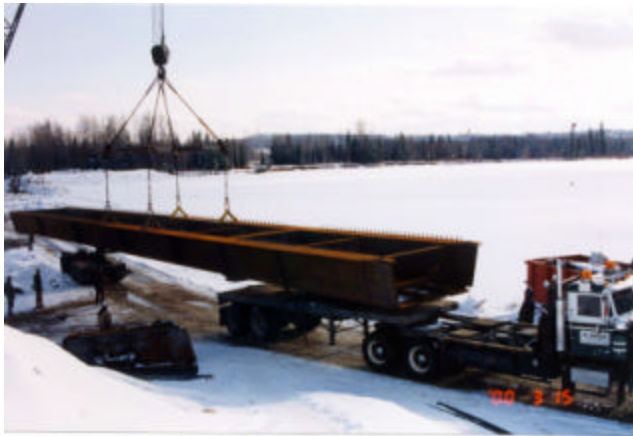
6-2 Spreader used to pick up box girder
