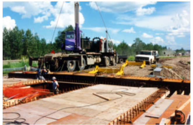
6-11 Deck joint installation
