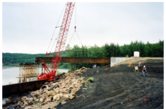
6-18 Erecting girder between abutment and temporary support tower at splice location
