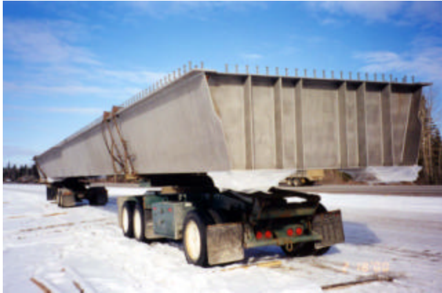
6-1 Trapezoidal box girder delivered with pot bearing assemblies attached
