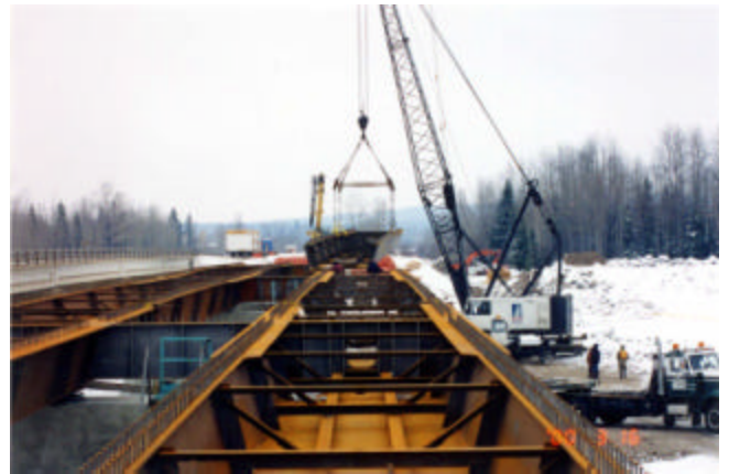
6-6 Girder erection in winter months utilizing single crane
