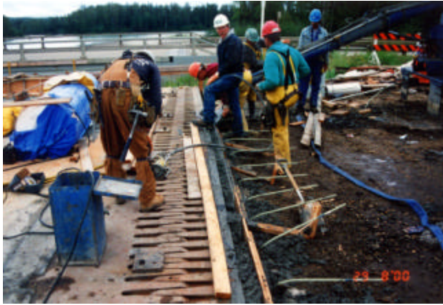
6-13 Casting in abutment side of finger plate deck joint
