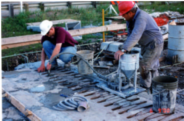
6-14 Pressure grouting voids under the finger plates
