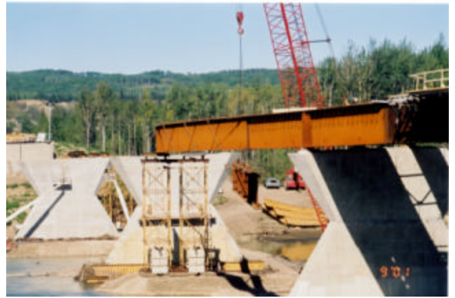
6-23 Girder erection between piers
