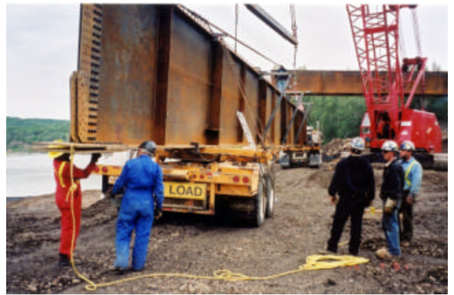
6-17 Girder delivered to site by truck
