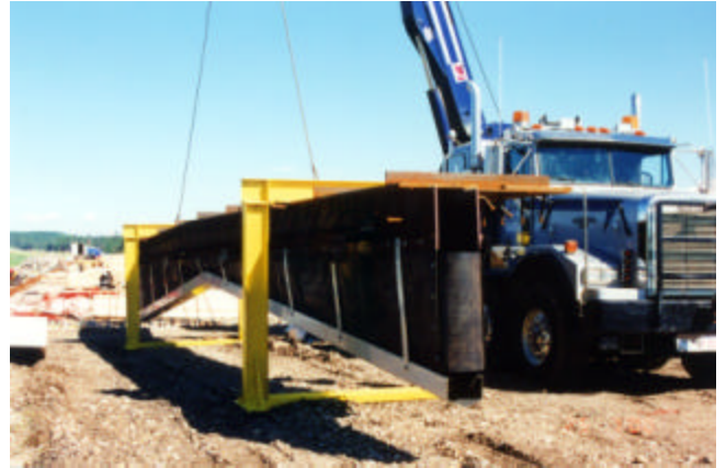
6-10 Finger plate deck joint assembly, delivery and temporary storage
