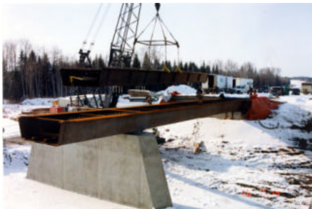
6-3 Erecting box girder between abutment and spanning over pier
