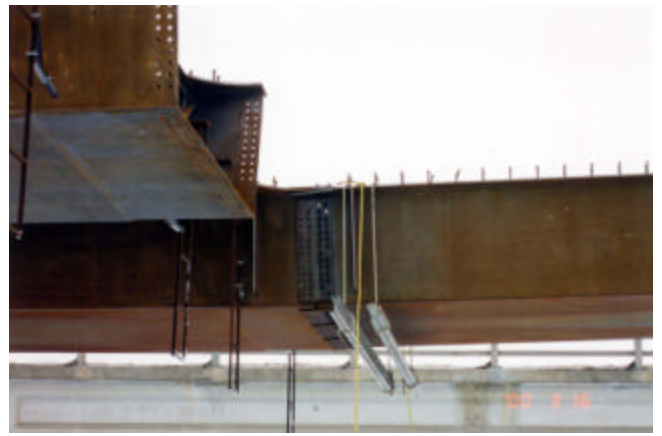
6-5 Splice connection between girder segments
