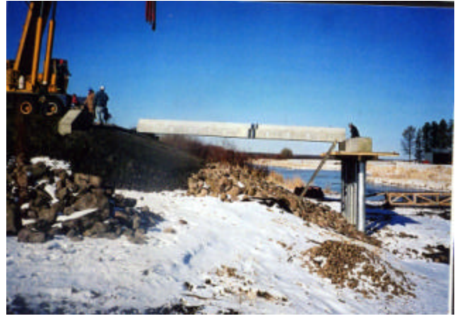
7-10 Erecting first span girders from approach
