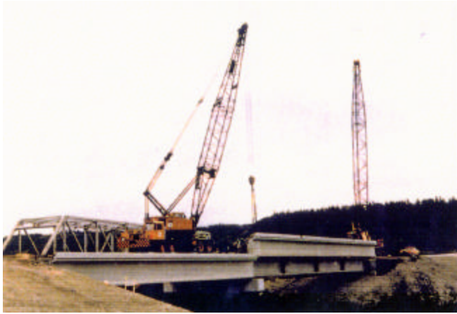
7-7 Erecting girders on top of previously erected girders
