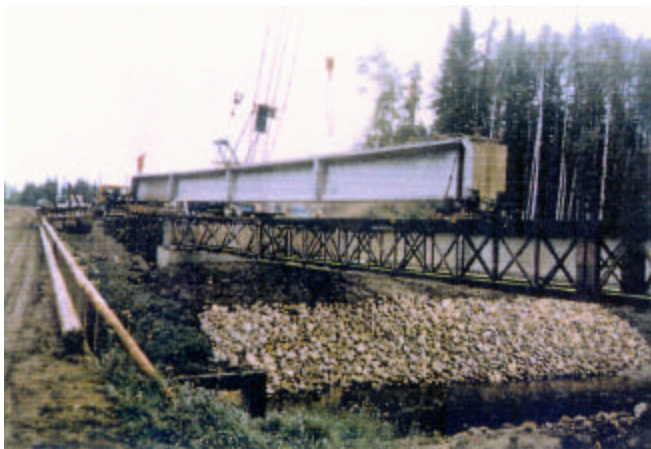
7-9 Using a launching truss for girder erection
