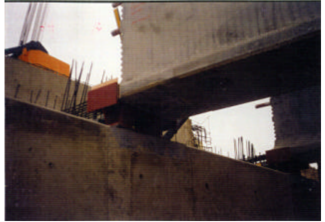
7-4 Girder on temporary bearing at abutment
