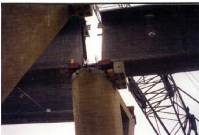
7-3 Girder on temporary bearing at pier
