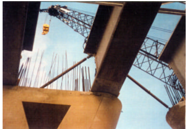
7-5 First girder erected, stabilized with temporary shoring
