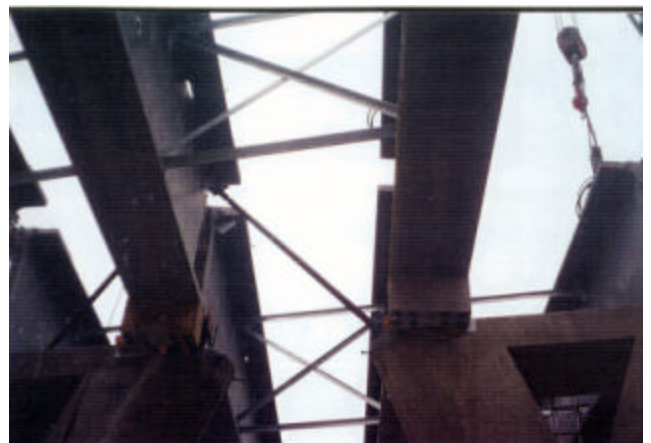
7-6 Subsequent girders erected, stabilized with permanent steel diaphragms
