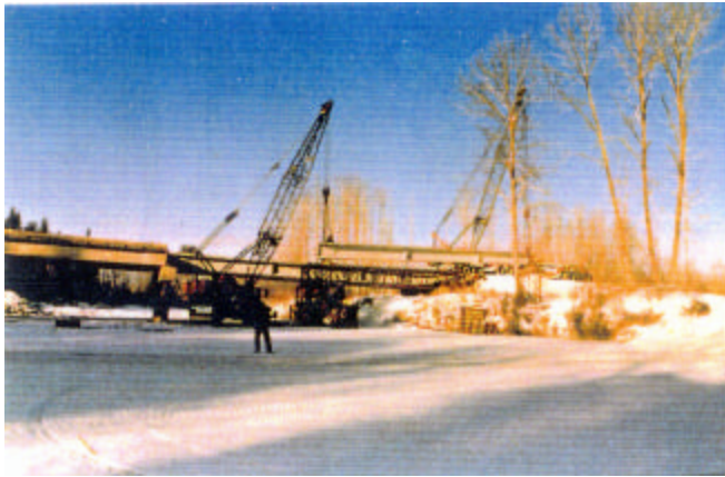
7-8. Erecting girders from the ice
