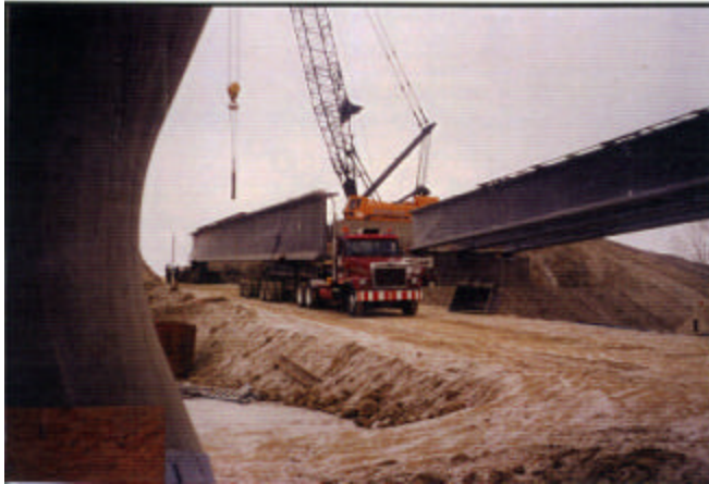
7-1 Precast concrete girder delivered to site
