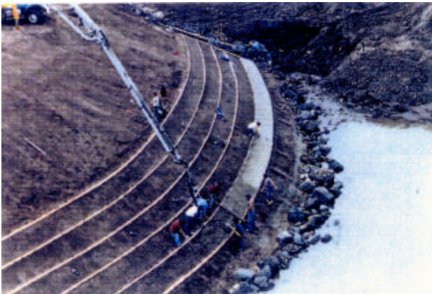
8-2 Horizontal strip concrete placement
