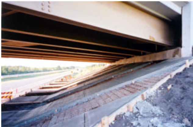
8-9 1st alternate vertical strip concrete placement complete
