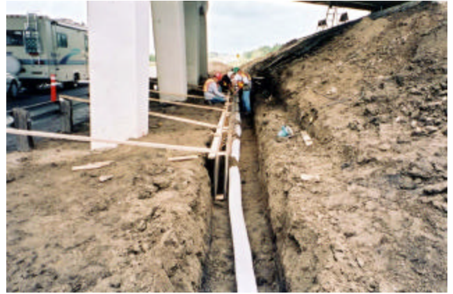
8-10 Forming key at the bottom of headslope
