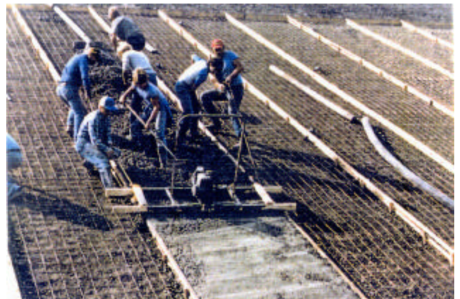
8-5 Vertical strip concrete placement
