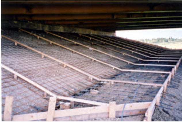
8-7 Formwork for upper concrete slope protection
