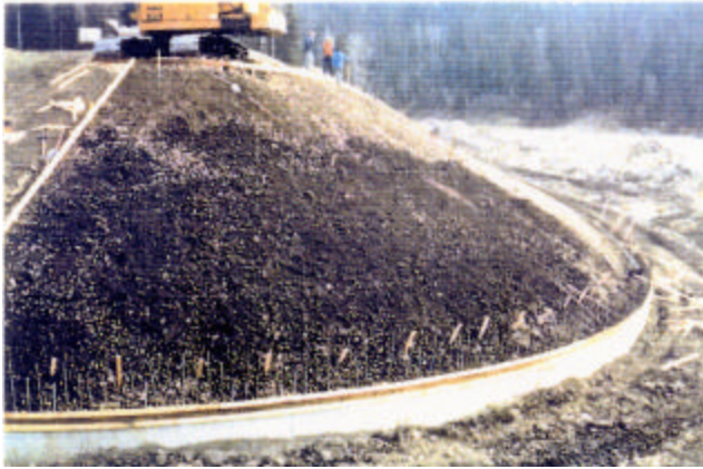
8-1 Preparation of headslope
