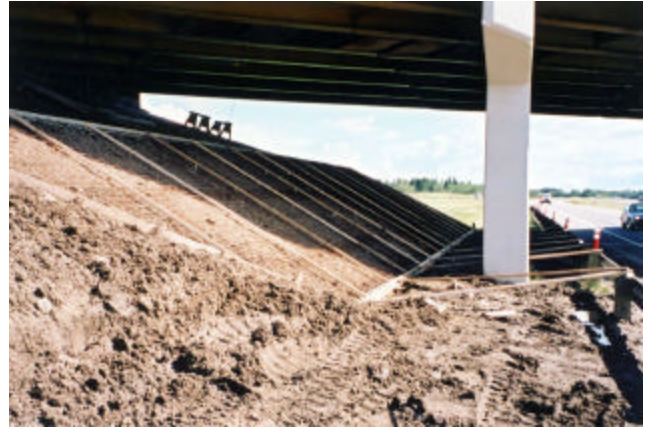
8-11 Formwork for lower half of concrete slope protection
