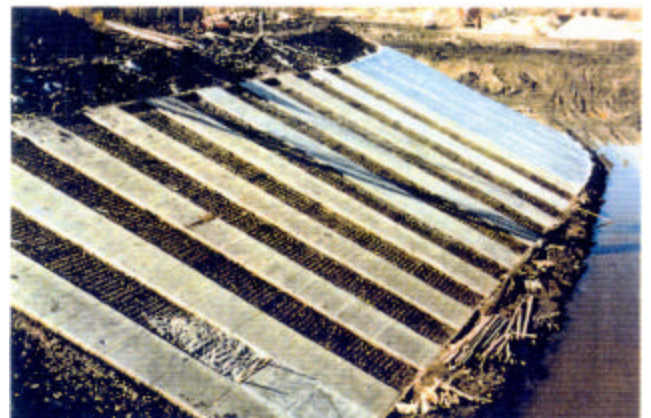
8-6 Pouring alternate vertical strips
