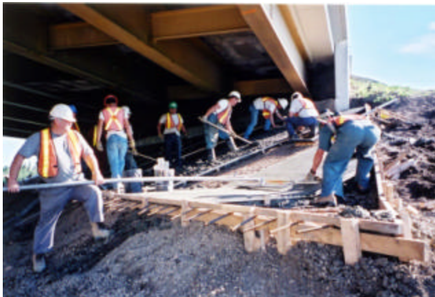
8-8 Alternate vertical strip concrete placement
