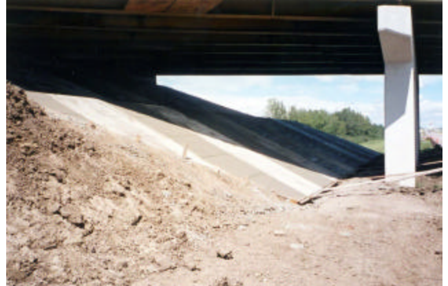
8-12 Concrete slope protection complete for lower portion
