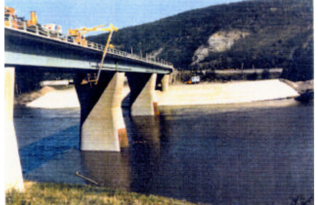
8-4 Concrete Slope Protection on headslope
