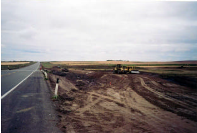
D-1 Construction of onsite detour
