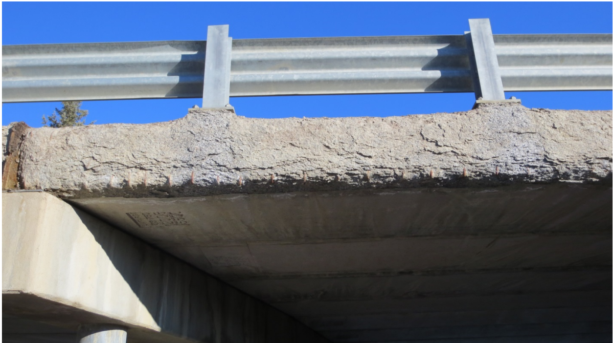
Example 4: Significant concrete section loss with exposed steel stirrups. Exterior girder rated 2. Concrete section loss extending below bridgerail post baseplate. Bridgerail posts rated 2.
