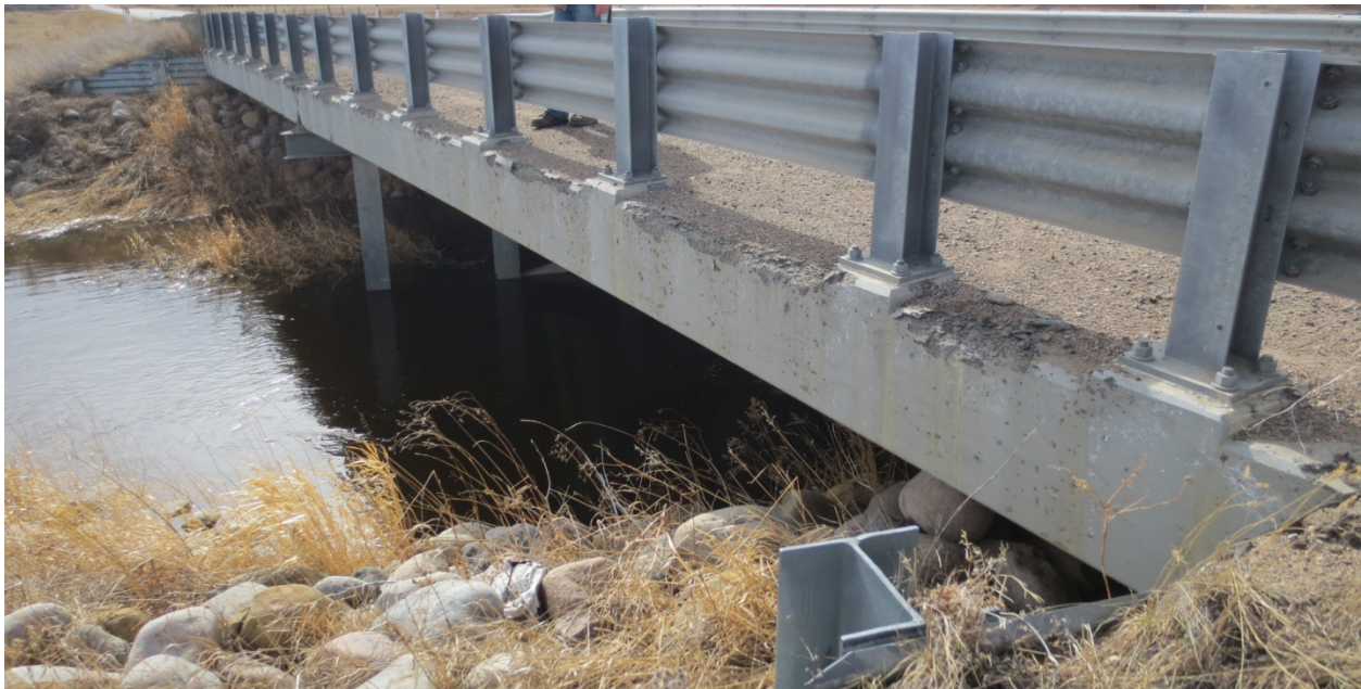
Example 5: Concrete section loss of exterior girder extending less than 50 mm from the top edge of the girder. Girder rated 3. Concrete section loss of bridgerail post plinth not extending to bridgerail post baseplate. Bridgerail post rated 3.
