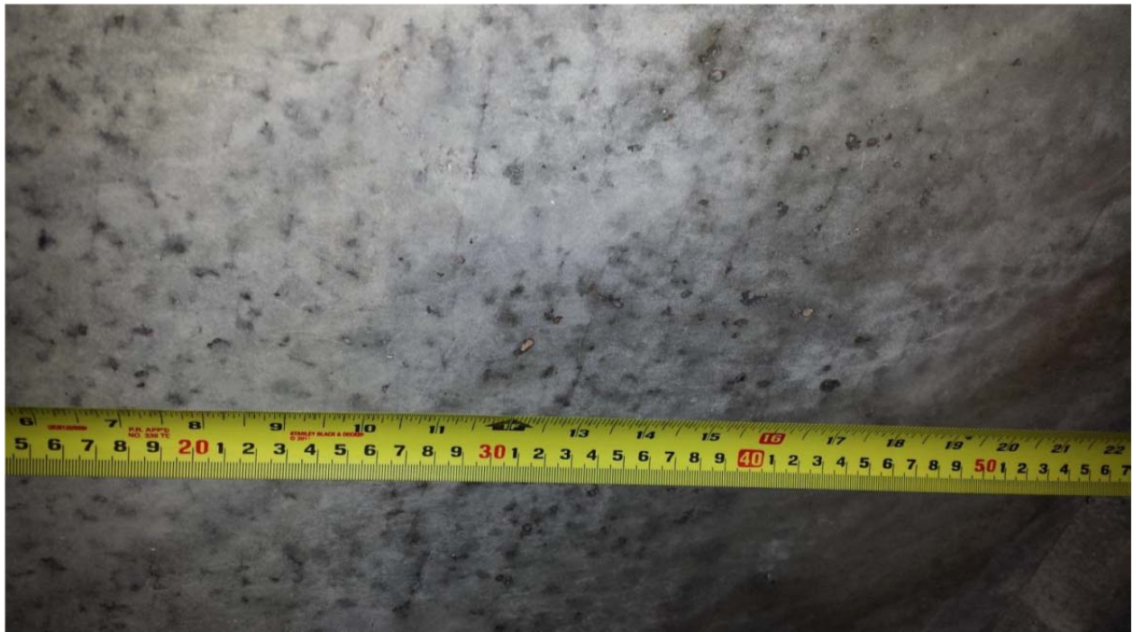
Example 7: Isolated aggregate popouts along interior girder. Girder rated 4.
