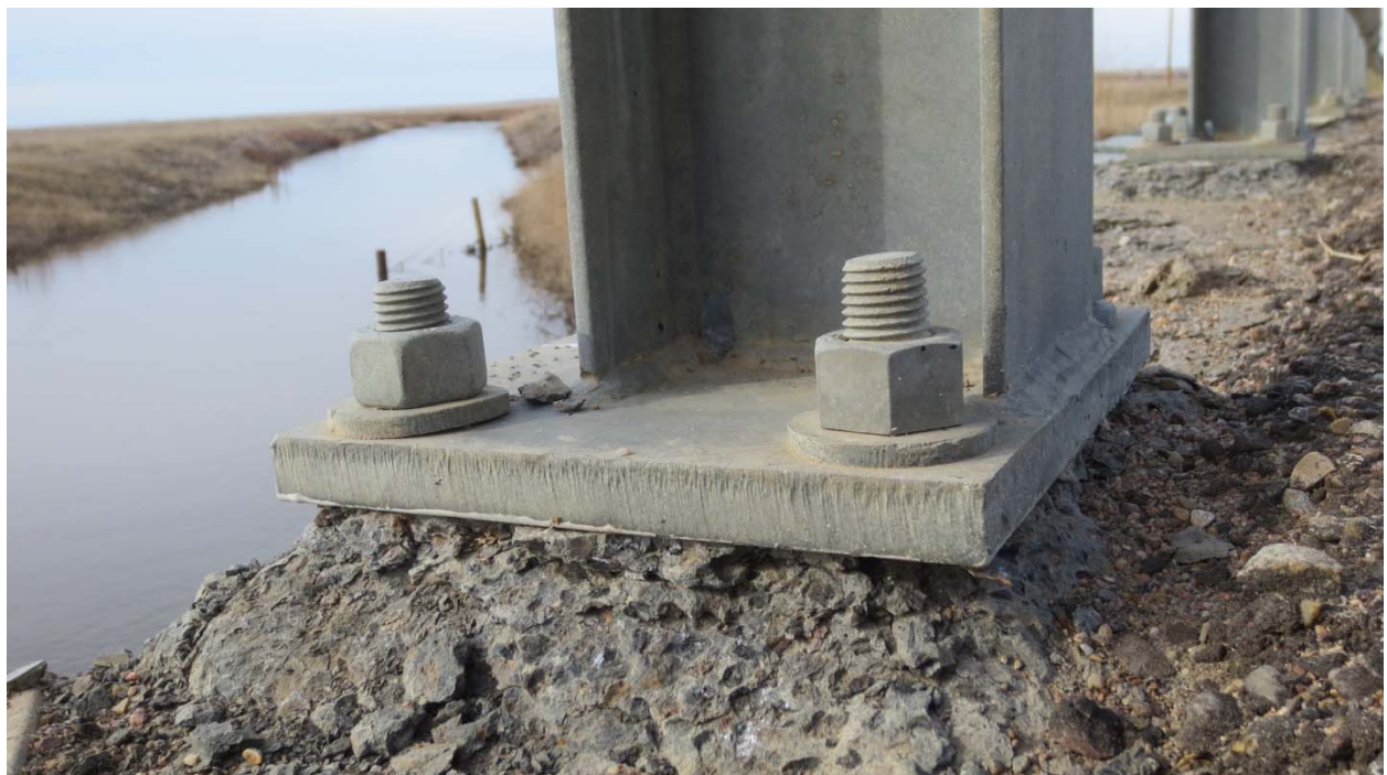
Example 8: Concrete plinth section loss extending below bridge rail base plate. Bridge rail post rated 2.
