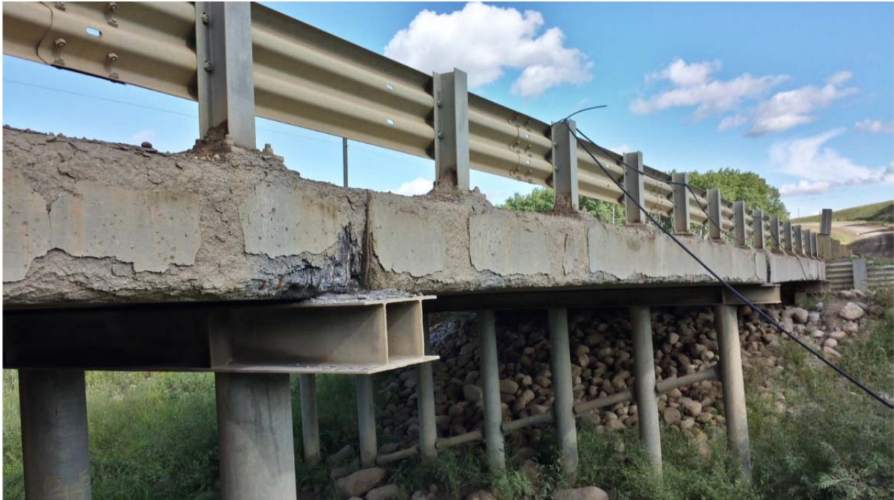
Example 1: Extensive scaling of exterior girder surfaces with concrete section loss extending more than 50 mm from top, bottom, and end edges of the girder. Exposed strand and stirrups. Concrete section loss of girder top that extends up to the edge of the bridge rail base plate. Girders rated 2. Bridge rail posts rated 2.
