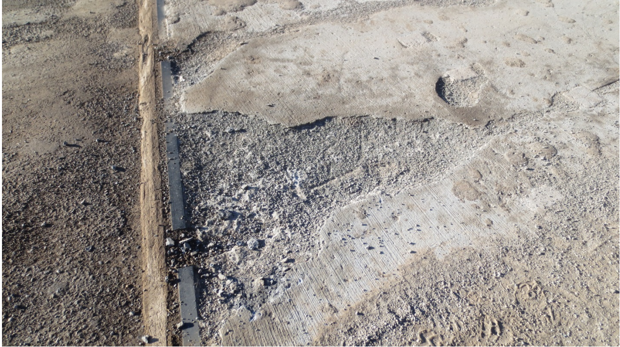
Example 3: Concrete section loss less than 35 mm in depth along top surfaces of interior girders. Interior girders rated 3.
