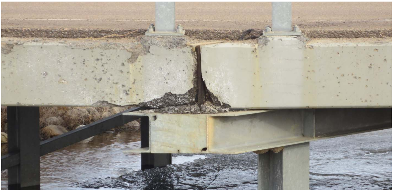
Example 6: Concrete section loss of exterior girder extending more than 50 mm from the vertical edge of the girder end. Girder rated 2. Concrete section loss of bridgerail post plinth extending to bridgerail post baseplate. Bridgerail post rated 2.
