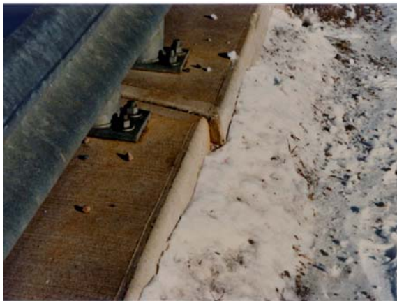
Figure 7.31 - Horizontal Misalignment
