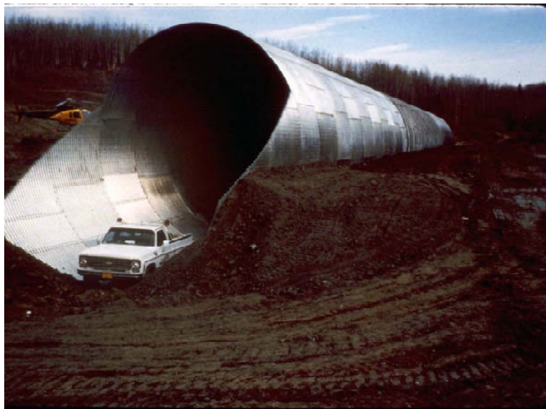
Figure 13.2 - Backfill of SPCSP Culvert
