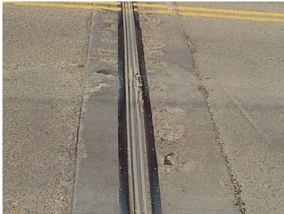
Figure 7.5 - Gland Joint
