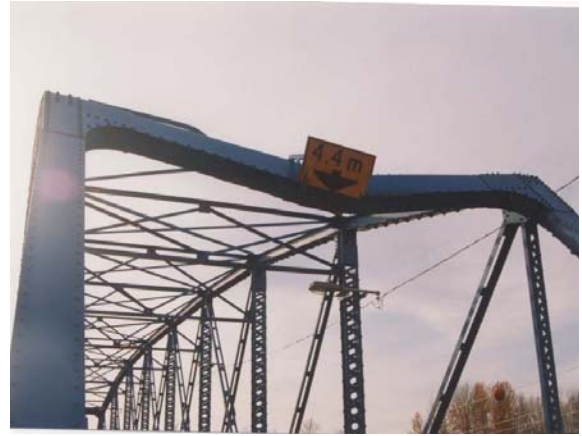
Figure 7.24 - Damaged Portal Bracing
