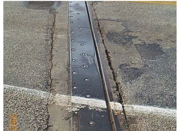
Figure 7.6 - Armoured Gland Joint
