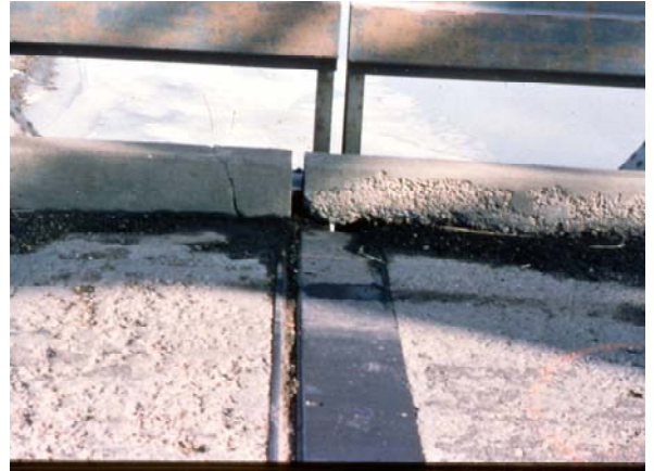
Figure 7.4 - Sliding Plate Joint
