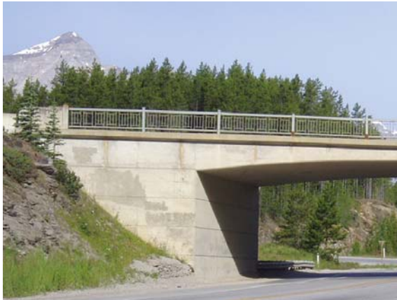
Figure 8.1 - Full Height Abutment
