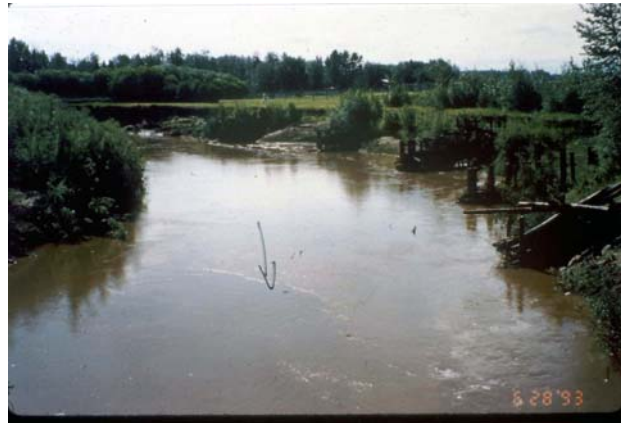
Figure 9.3 - Timber Crib Spurs
