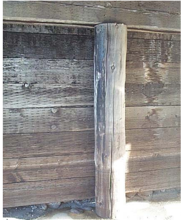
Figure 8.14 - Checks in Timber Pile
