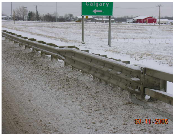
Figure 6.1 - Current Approach Rail Standard
