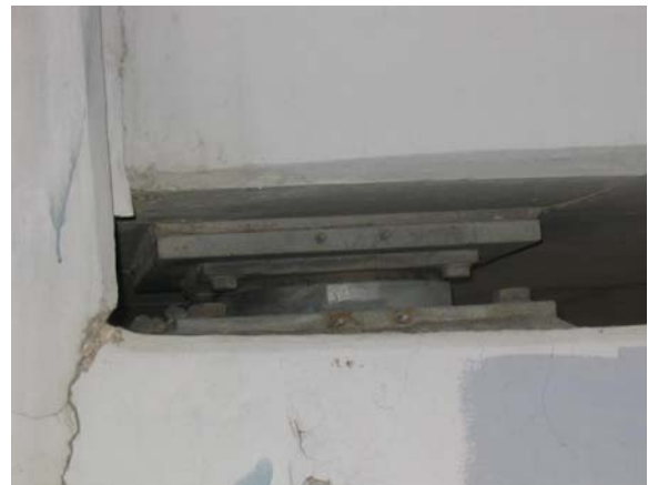
Figure 7.29 - Pot Bearing
