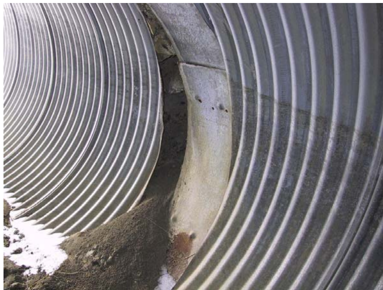
Figure 13.9 - Separated Circumferential Seam
