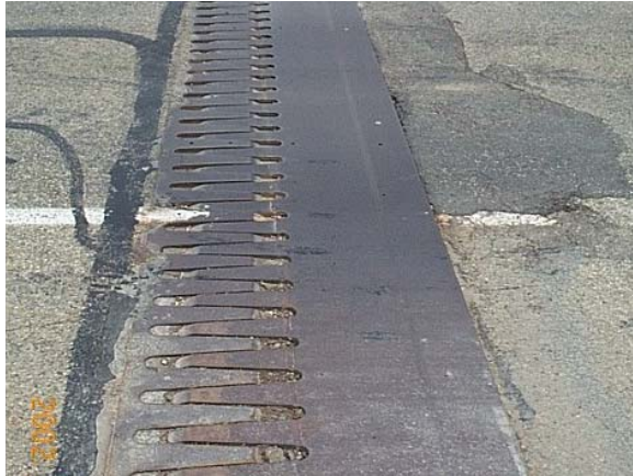
Figure 7.3 - Finger Plate Joint
