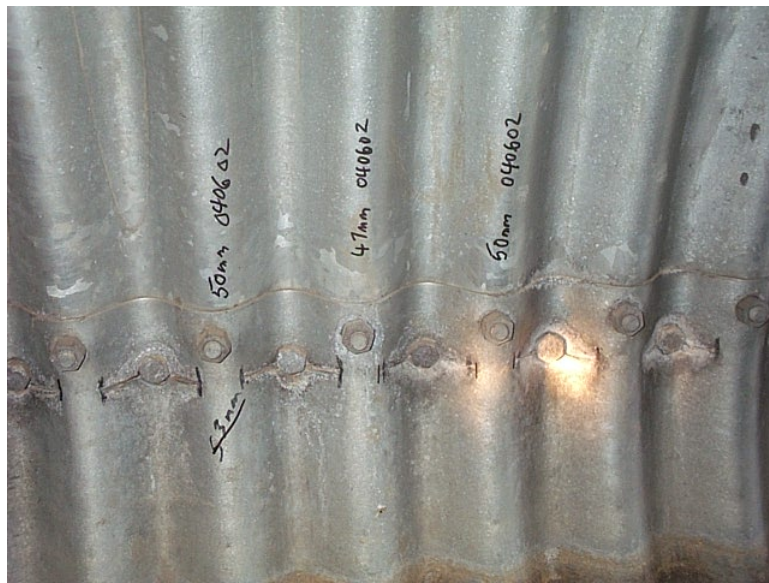
Figure 13.11 - Improperly Lapped Seam with Longitudinal Cracks
