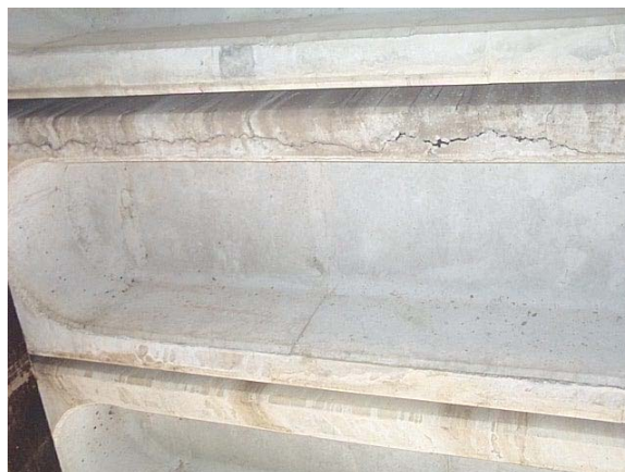
Figure 7.15 - Wide Crack in Anchorage Zone
