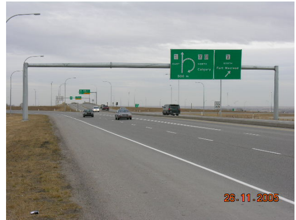
Figure 15.2 - Tube Type Sign Structure
