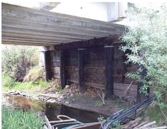
Figure 8.11 - Backwall Sheeting Needs Lowering
