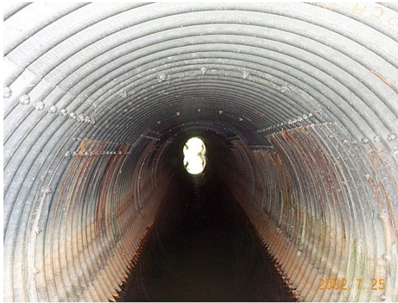
Figure 13.12 - Minor Corrosion, Rated 5
