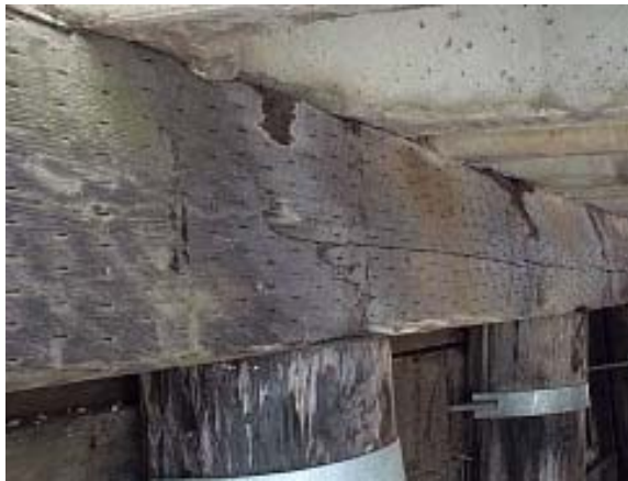
Figure 8.5 - Bulging of Timber Cap
