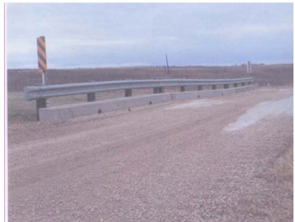
Figure 7.32 - Vertical Misalignment
