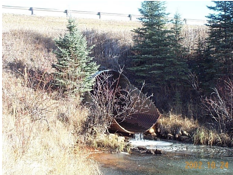
Figure 13.16 - Culvert with Hanging Invert
