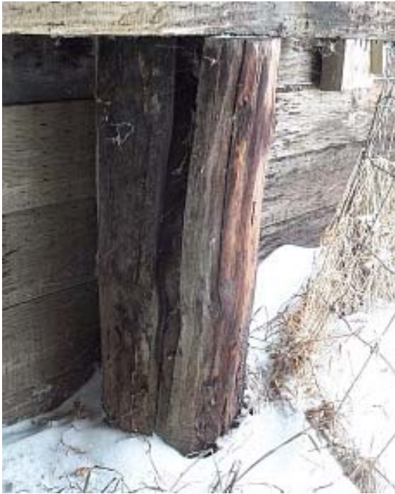
Figure 8.13 - Split Timber Pile
