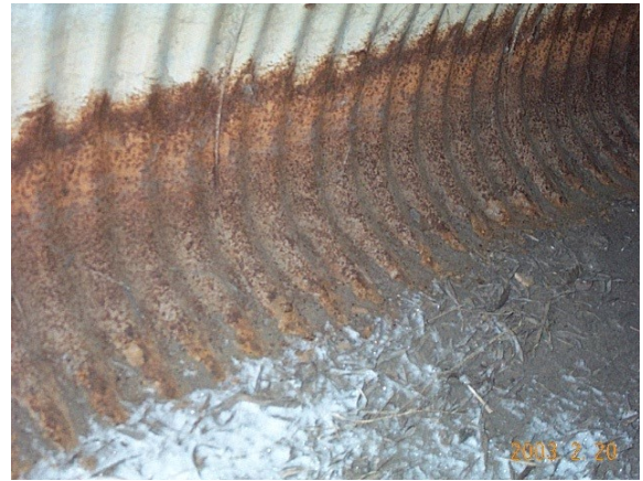
Figure 13.13 - Heavy Corrosion, Rated 4
