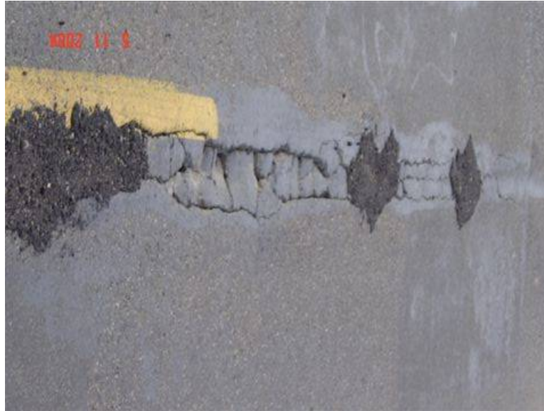
Figure 7.11 - Lateral Connection Failure
