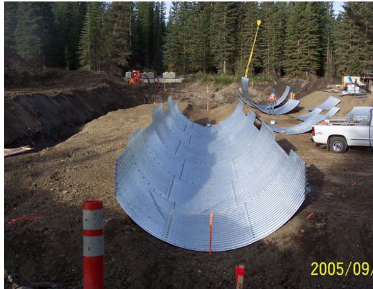
Figure 13.1 - Assembly of SPCSP Culvert
