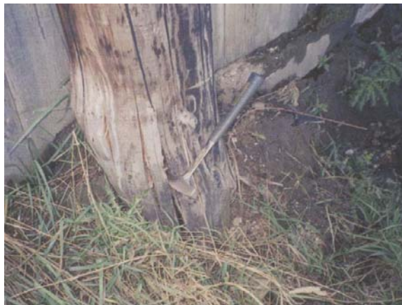
Figure 8.15 - Rot in Timber Pile
