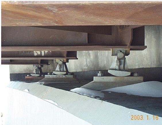
Figure 7.26 - Rocker Bearing
