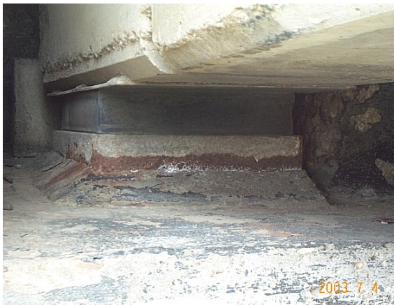
Figure 7.28 - Reinforced Neoprene Pad
