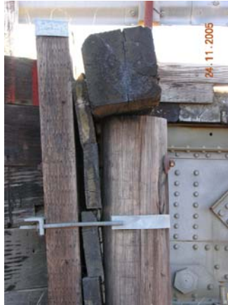
Figure 8.7 - Timber Cap Rotating
