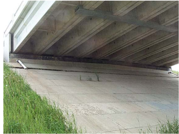
Figure 8.2 - Spill-through Abutment
