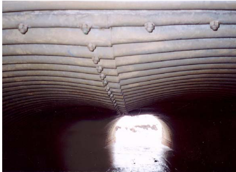
Figure 13.7 - Culvert Roof with Reverse Curvature
