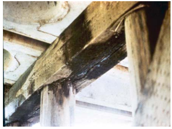
Figure 8.6 - Crushing of Timber Cap
