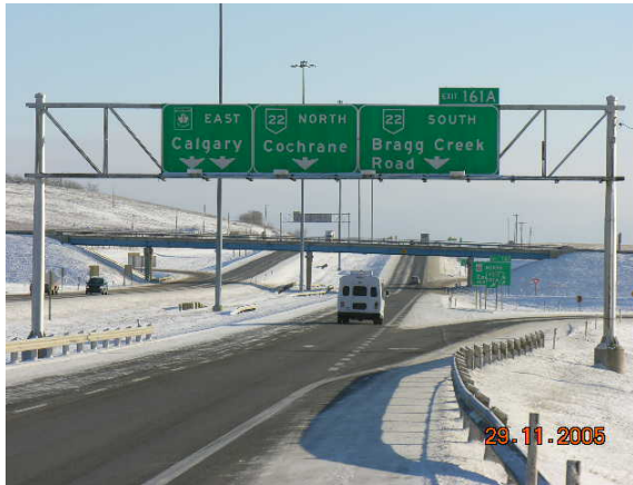
Figure 15.1 - Truss Type Sign Structure
