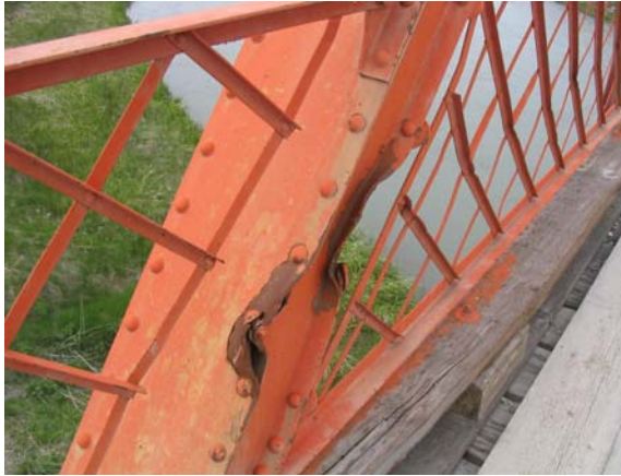
Figure 7.23 - Damaged Batter Post
