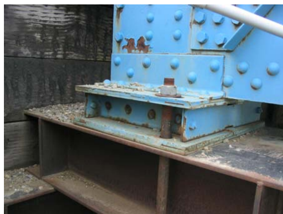
Figure 7.30 - Roller Nest Bearing
