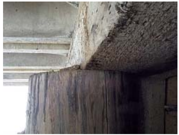
Figure 8.4 - Insufficient Bearing
