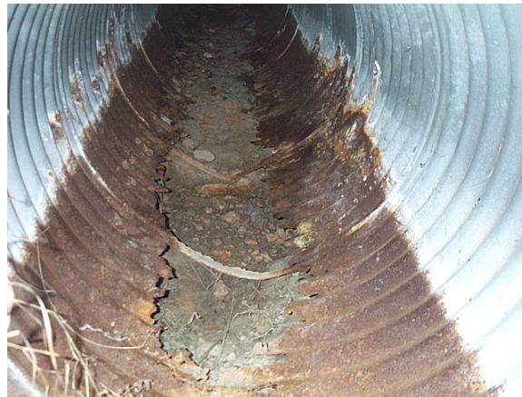
Figure 13.14 - Severe Corrosion, Rated 2
