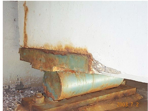
Figure 7.27 - Roller Bearing
