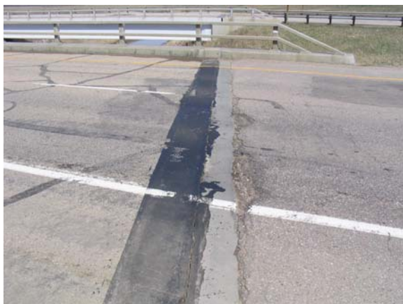
Figure 7.7 - Asphalt Plug Joint
