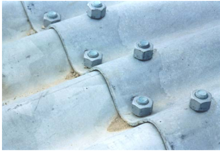
Figure 13.10 - Properly Lapped Seam
