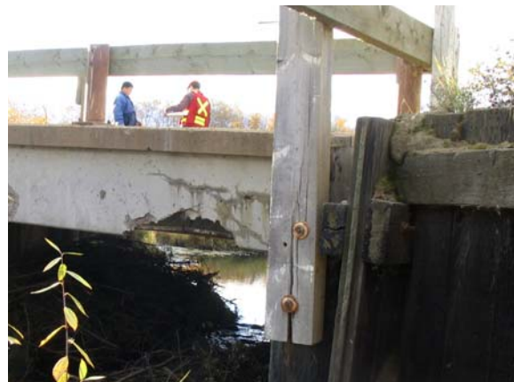
Figure 7.17 - Spall in Anchorage Zone with Unsound Concrete
