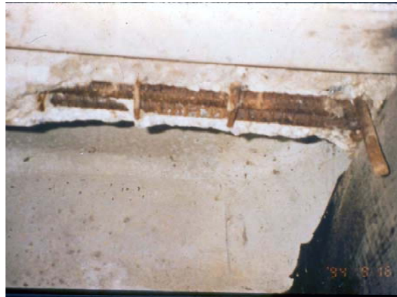
Figure 7.16 - Spall in Anchorage Zone with Sound Concrete
