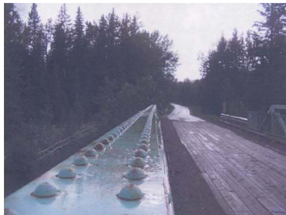
Figure 7.25 - Sweep in Top Chord
