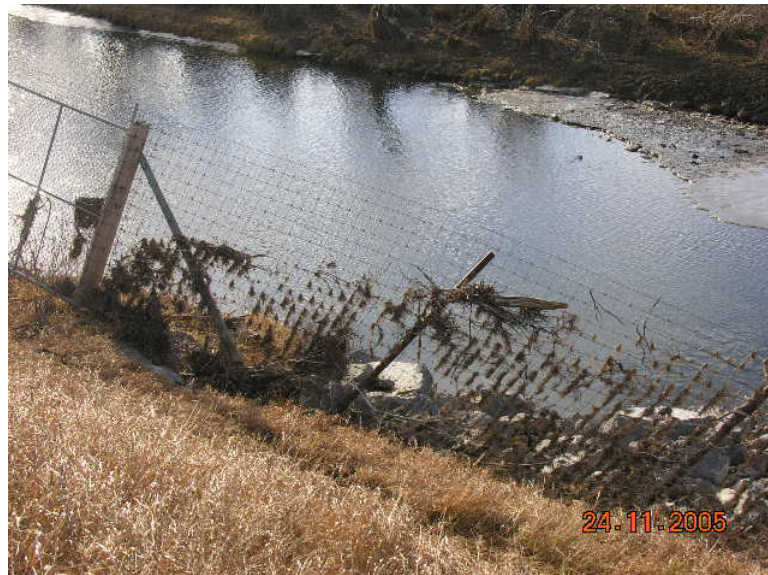
Figure 13.17 - Evidence of HWM
