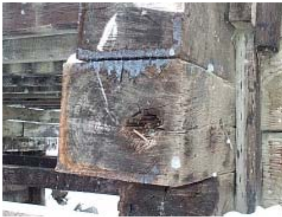
Figure 8.3 - Rot in Timber Cap
