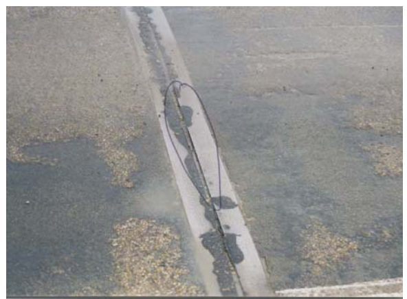
Figure 7.8 - Buffer Angle Joint
