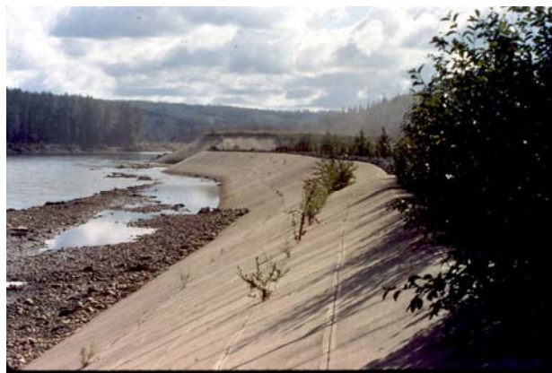
Figure 9.1 - Guidebank with Concrete Slope Protection
