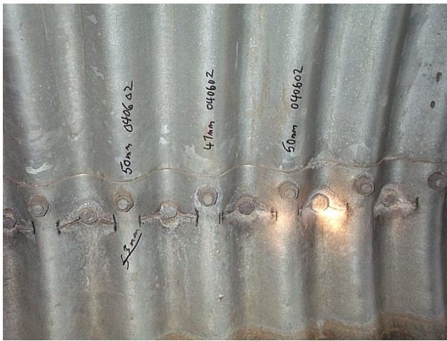
Figure 13.11 - Improperly Lapped Seam with Longitudinal Cracks
