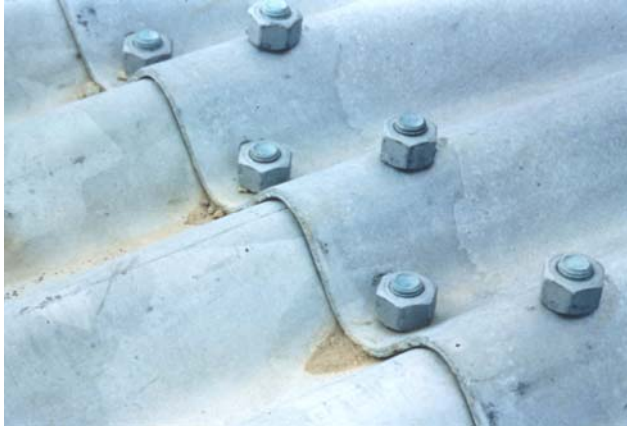
Figure 13.10 - Properly Lapped Seam
